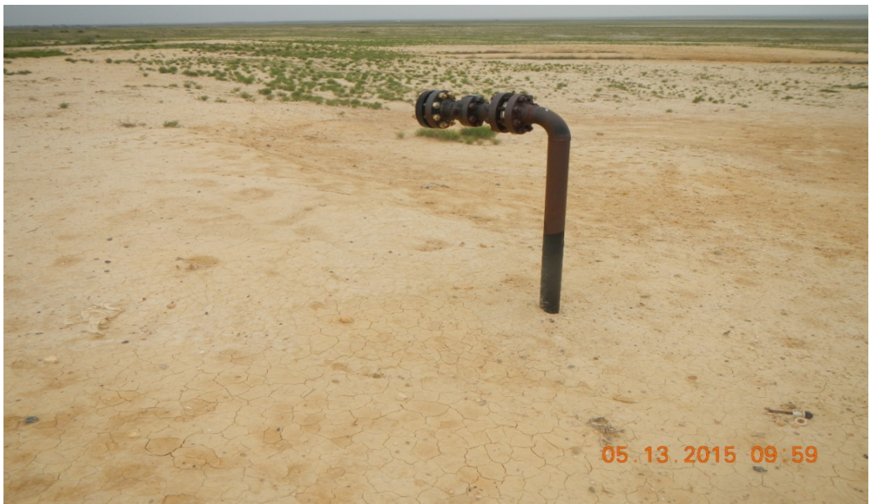
photo 4: Pipe riser remains on the location (Lat/Long: 38.38077, -102.69541).
