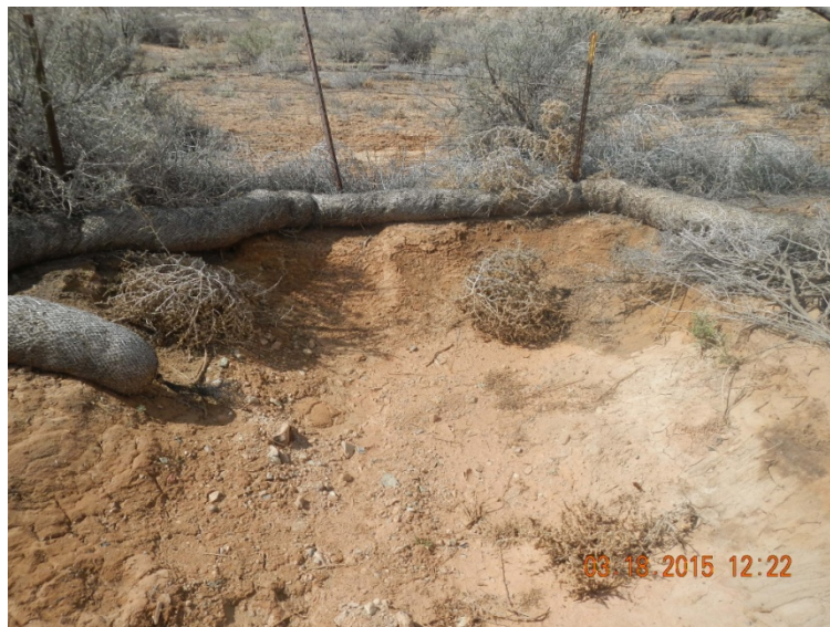
Furthest extent of spill #3 and excavated material. Material was stock piled on Monument Global Cache Unit #26 location. Per conversation with Tom Fox, material has been moved to tank battery across the valley to be land farmed.
