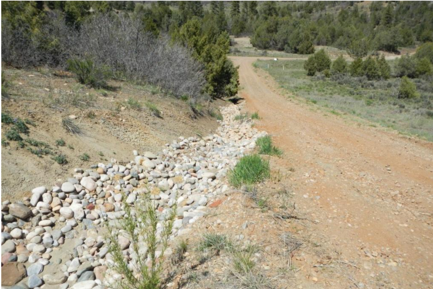
Photo 3. View of cobble lining along drainage adjacent to access road.
