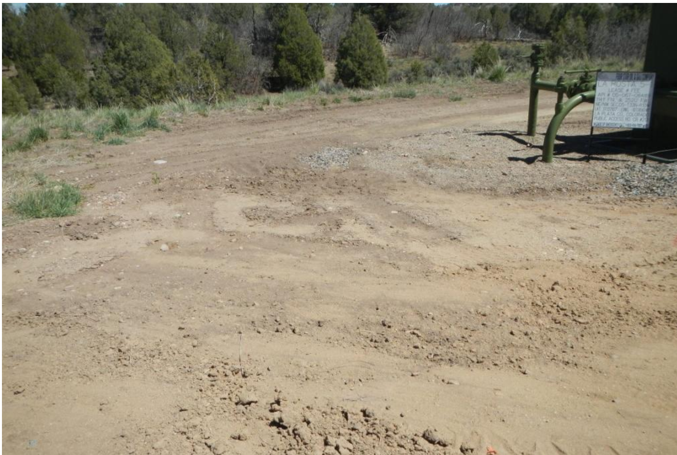
Photo 1. View of erosional feature that has been re-graded in northern portion of project area.
