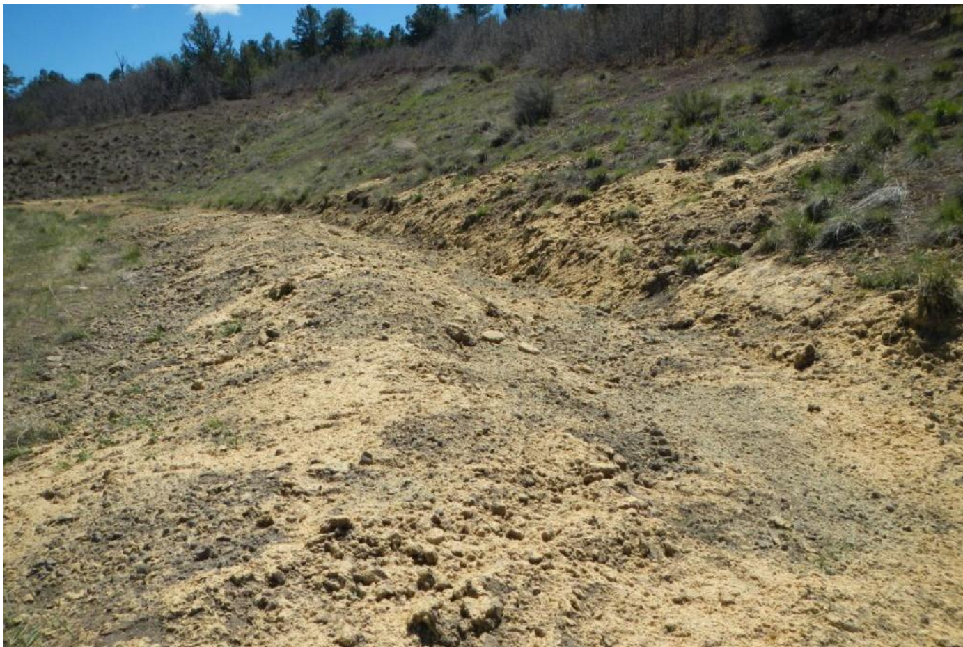
Photo 4. View of hydromulch on southern stormwater diversion channel and berm.
