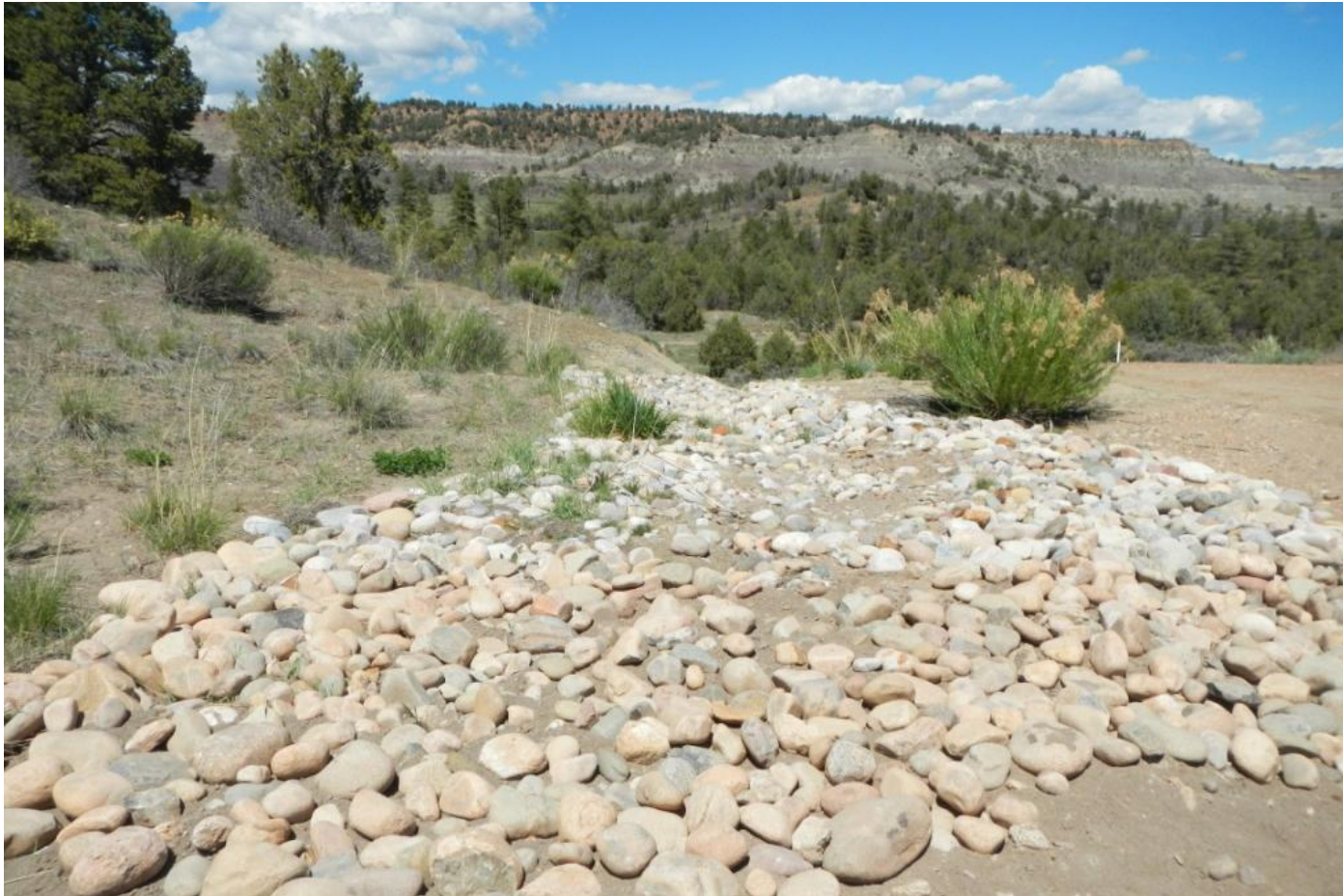
Photo 2. View of cobble on well pad surface where it appears that concentrated stormwater flows exit the project area.
