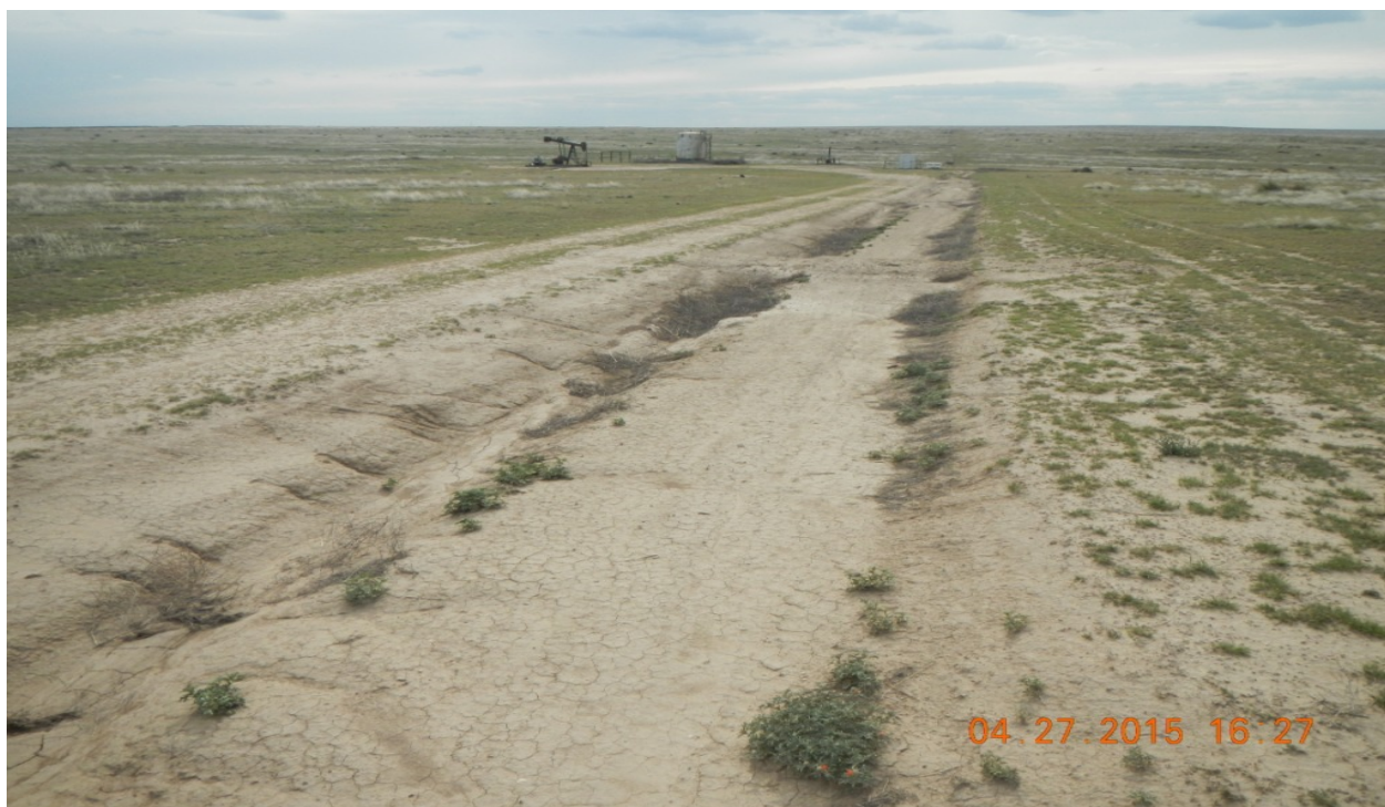
photo 4: Erosion along the old access road has caused vehicle traffic to widen the road to approx. 50 ft.
