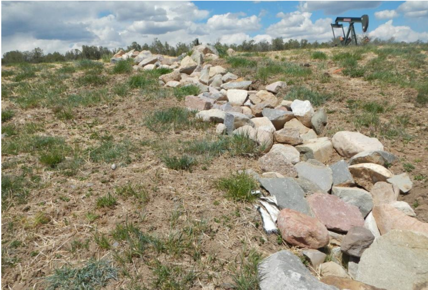
Photo 5. View of stormwater BMP and vegetation along southern slope of project area. These appear to be helping stabilize the location.
