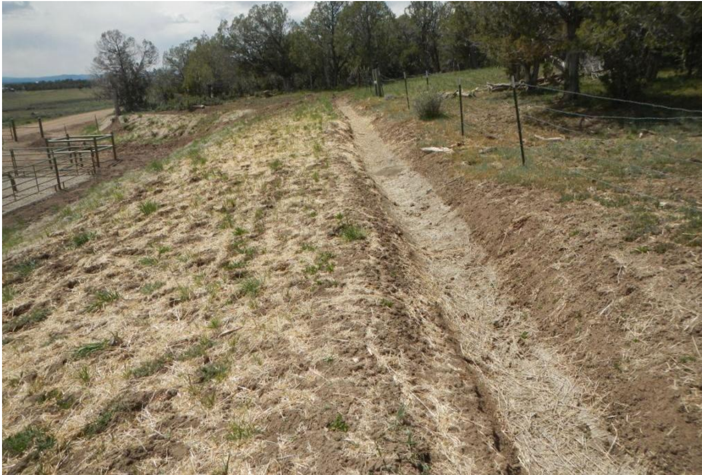
Photo 6. View of stormwater diversion drainage with straw blanket along northern edge of project area facing westward.
