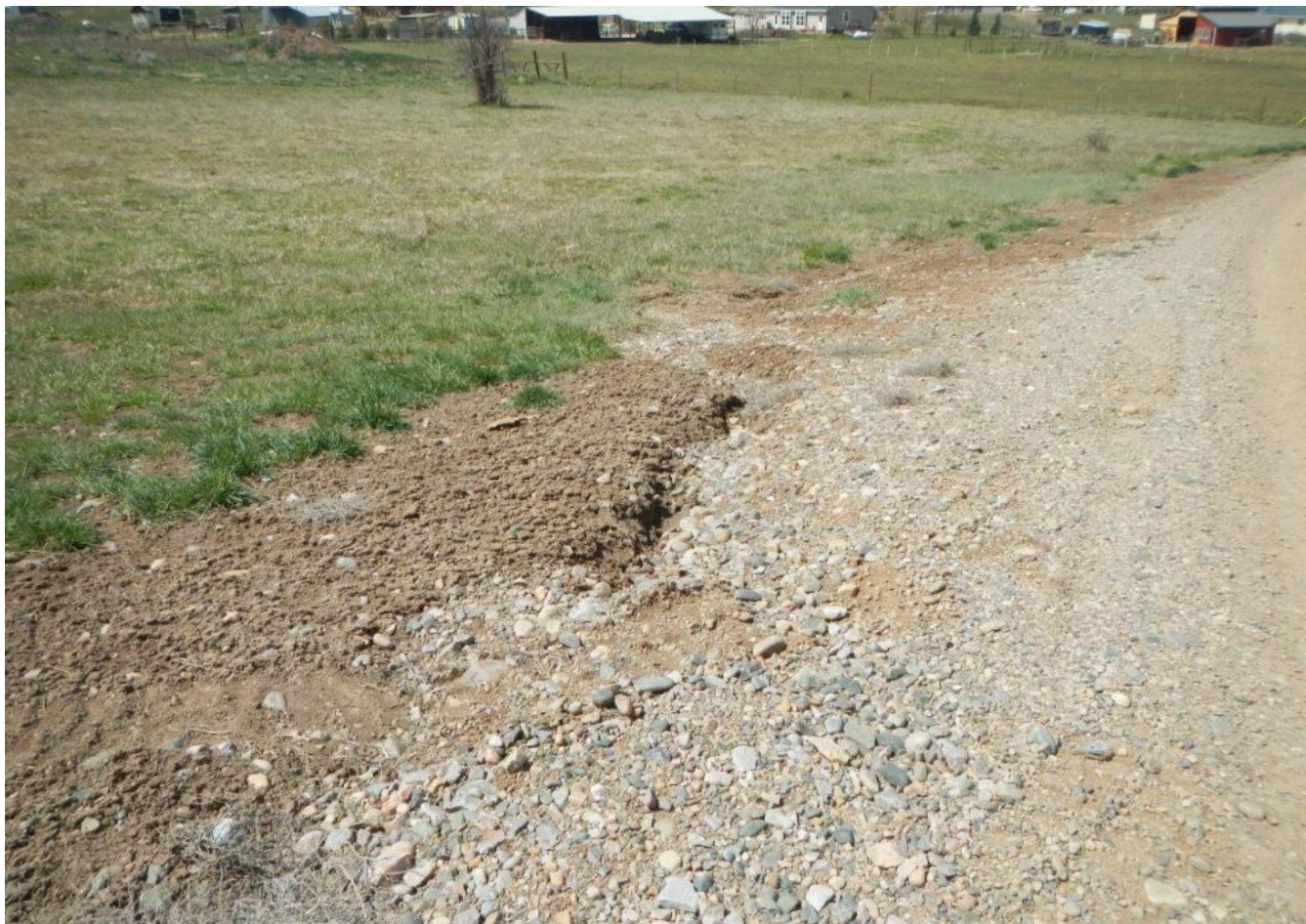
Photo 1. View of rill erosion coming off of access road that needs to be monitored.
