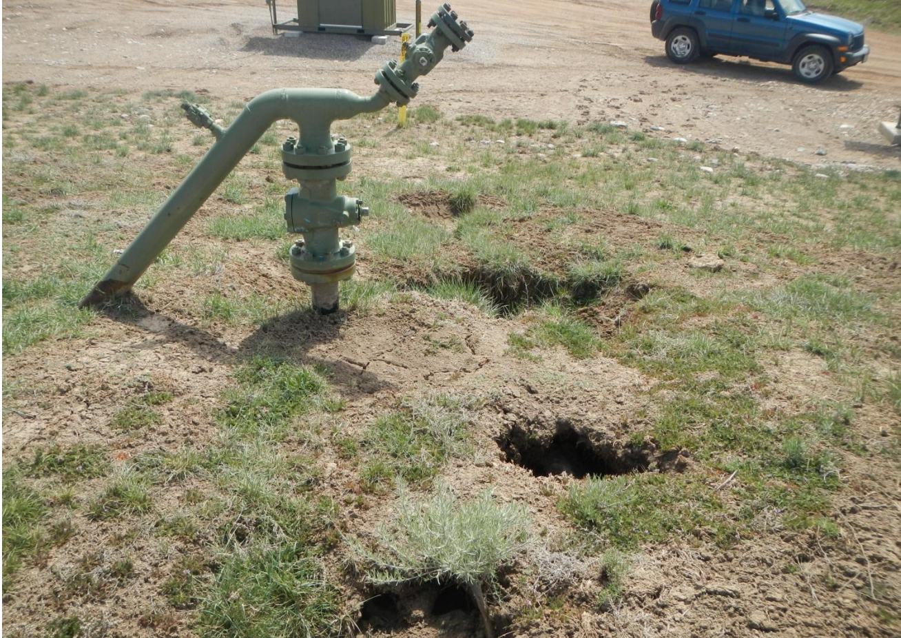
Photo 3. View of erosional channel tunneling beneath the northern portion of the interim reclamation area.
