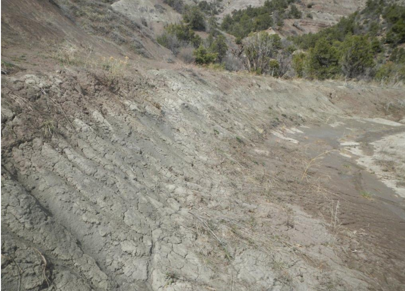
Photo 2. View of erosion along cut-slopes on western edge of project area.
