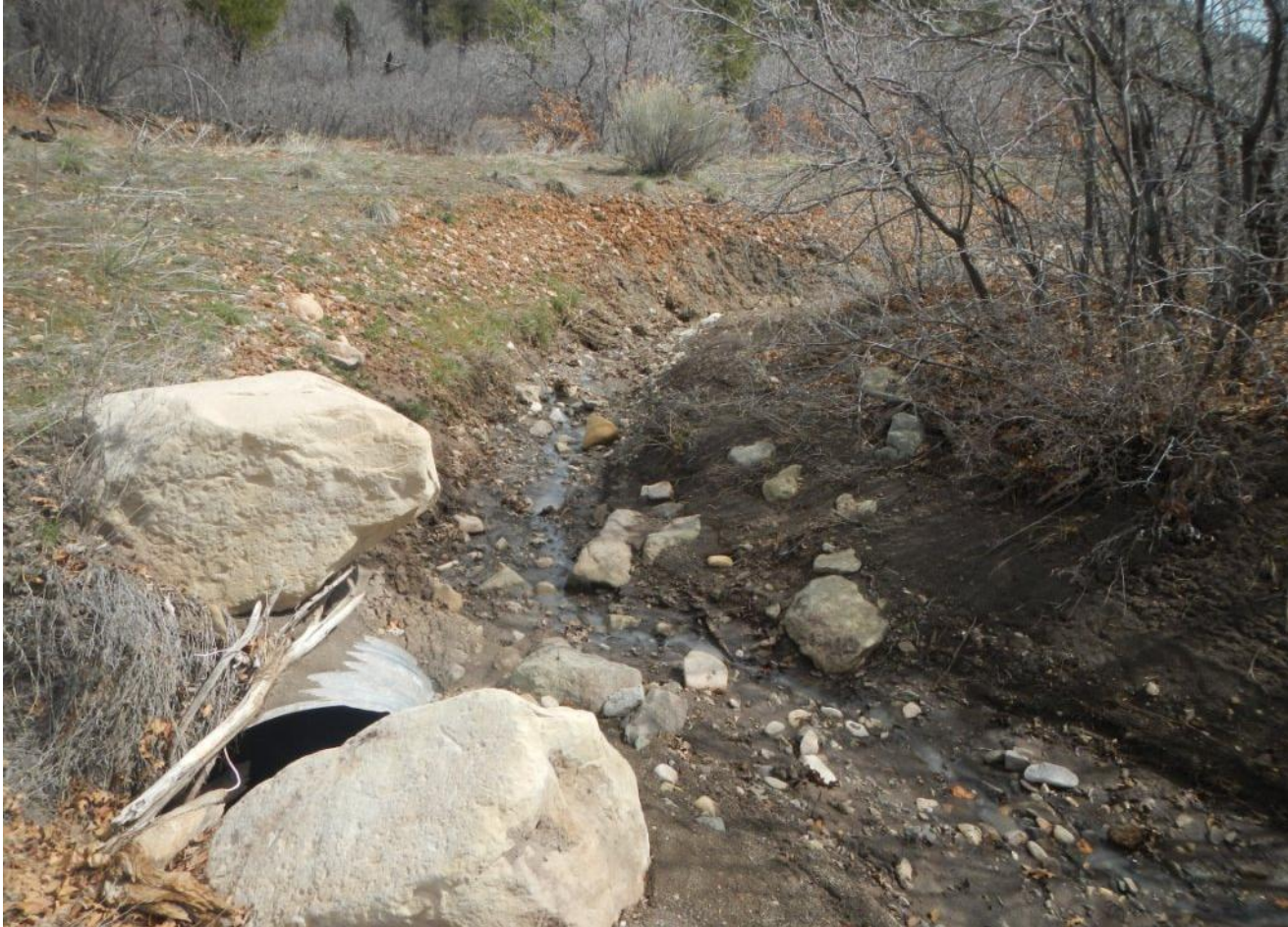
Photo 7. View of culvert inlet near the entrance to the well pad. It appears that a boulder has blocked the culvert and diverted the stream along the access road for approximately 700 feet.
