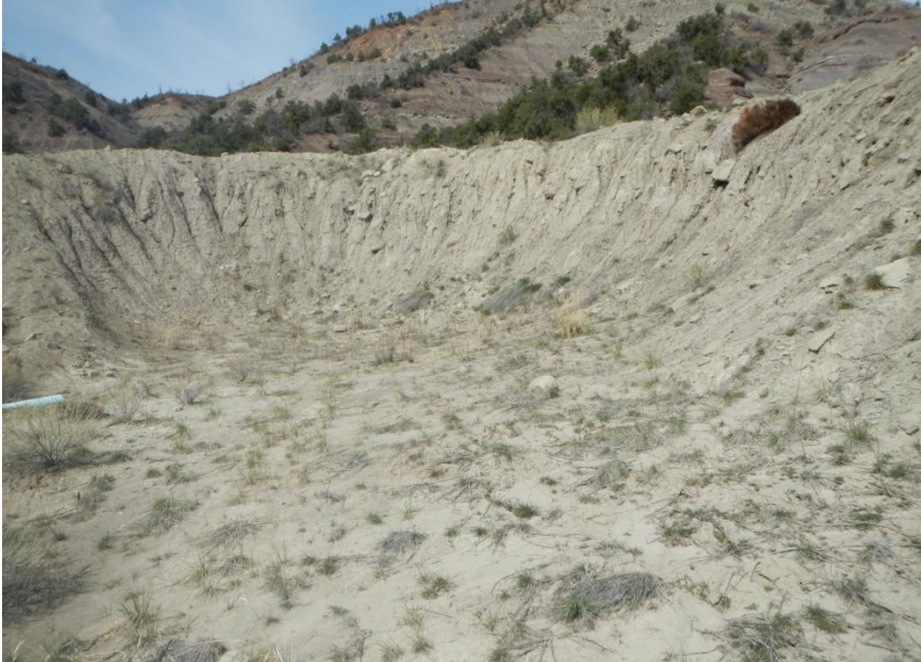
Photo 3. View of erosion of stockpiled soil in northwestern corner of project area.
