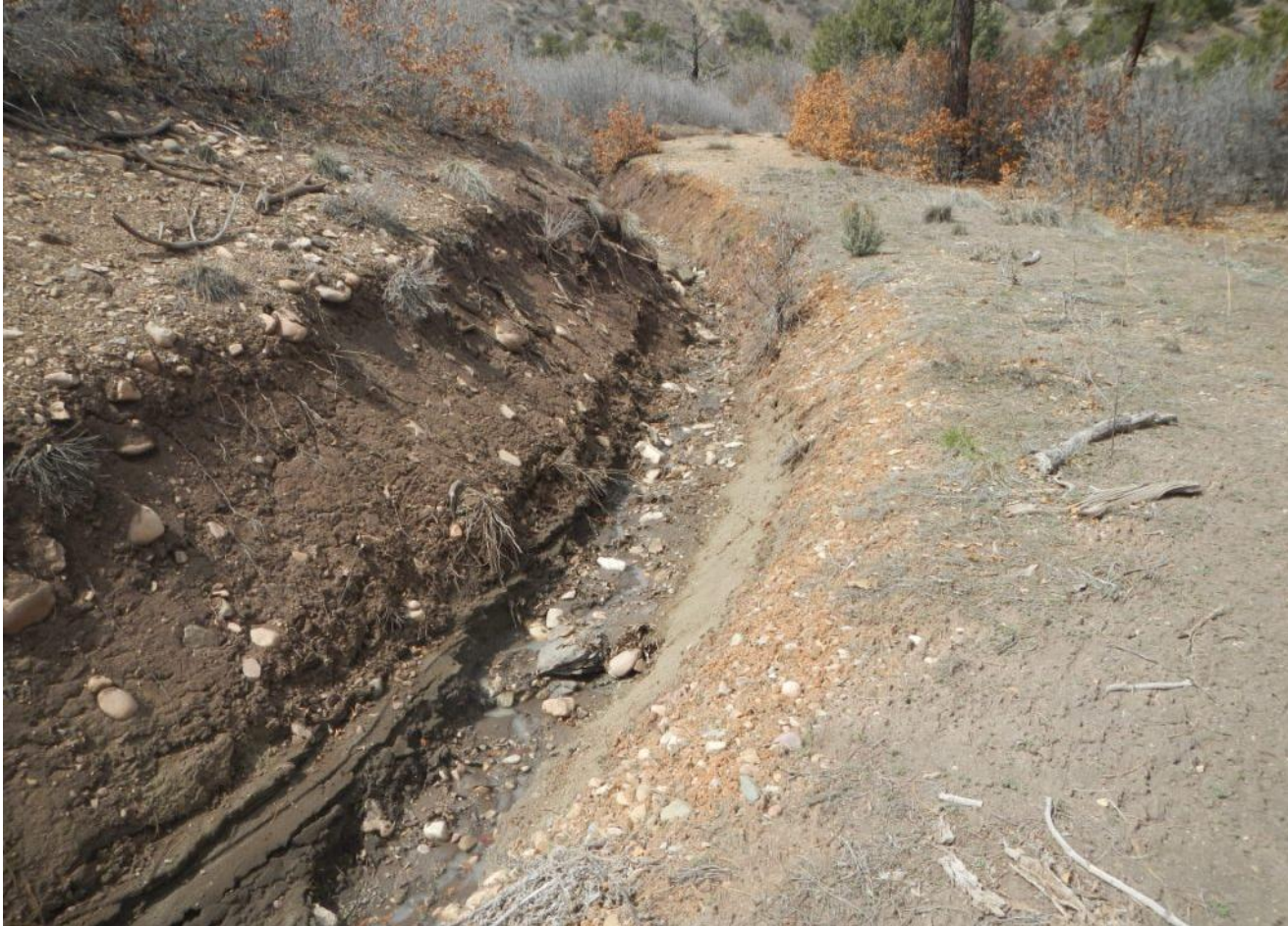
Photo 8. View of erosional channel approximately 3 to 6 feet wide and 2 to 5 feet deep along access road.
