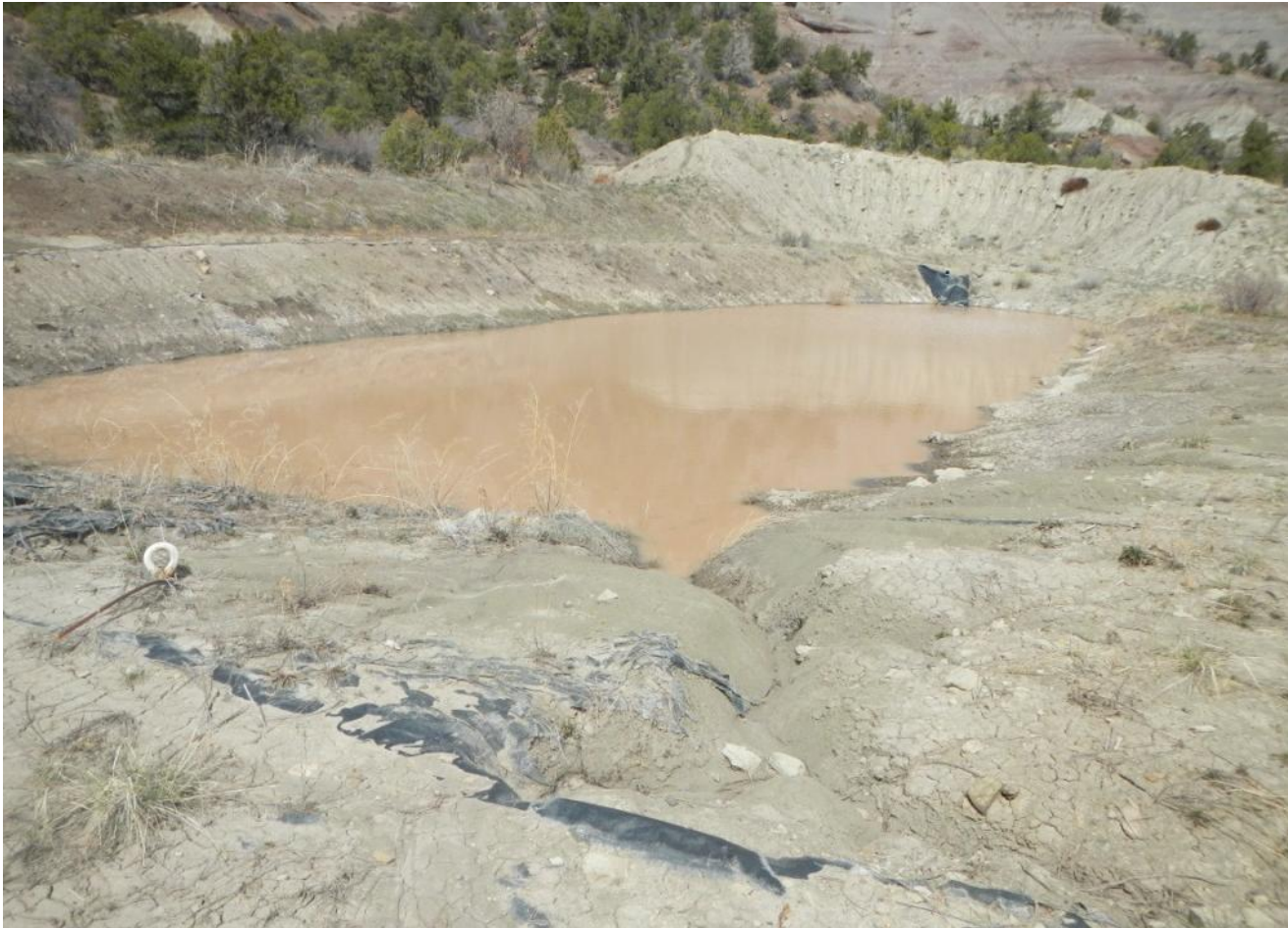
Photo 1. View of existing pit, pit liner, rig anchor, and sediment deposition on the well pad, facing northwestward.
