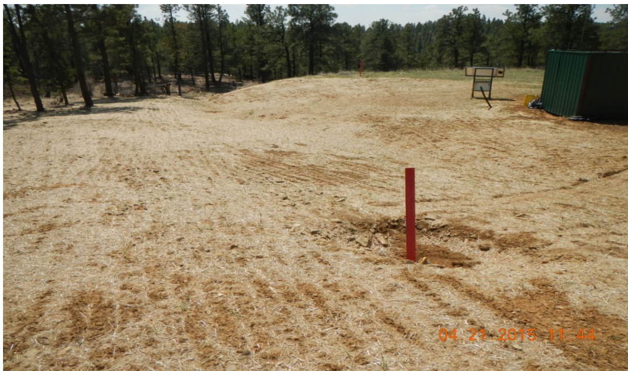
photo 4: : East side of the location has recently been seeded/mulched.
