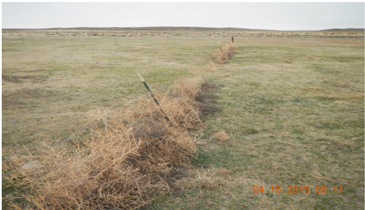
photo 8: Fence around the location is down at several places. Weed debris in fence.
