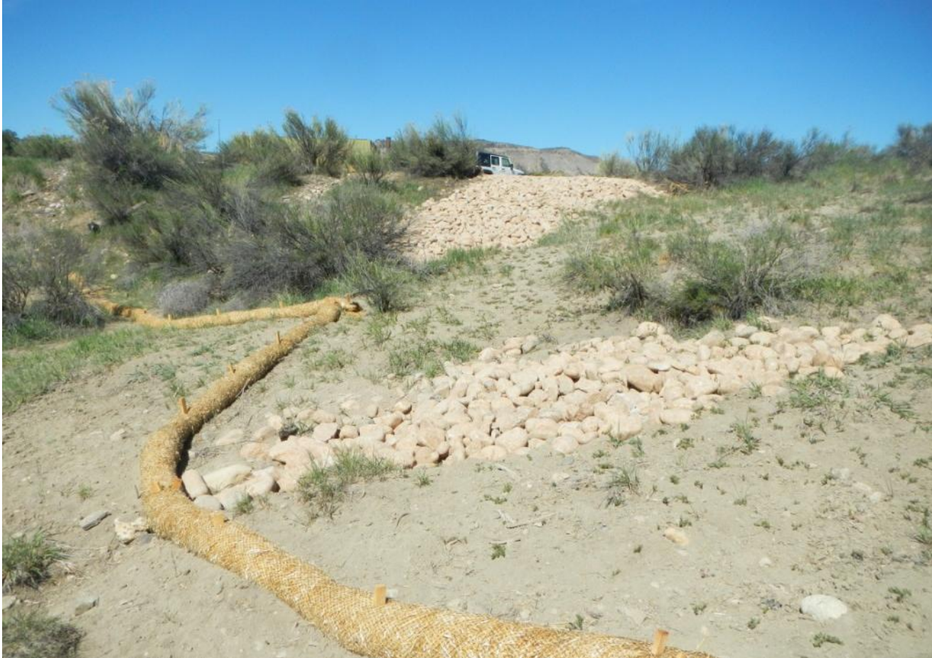
Photo 4. View of new stormwater BMPs installed within the eastern portion of the project area facing northwestward toward the well pad.
