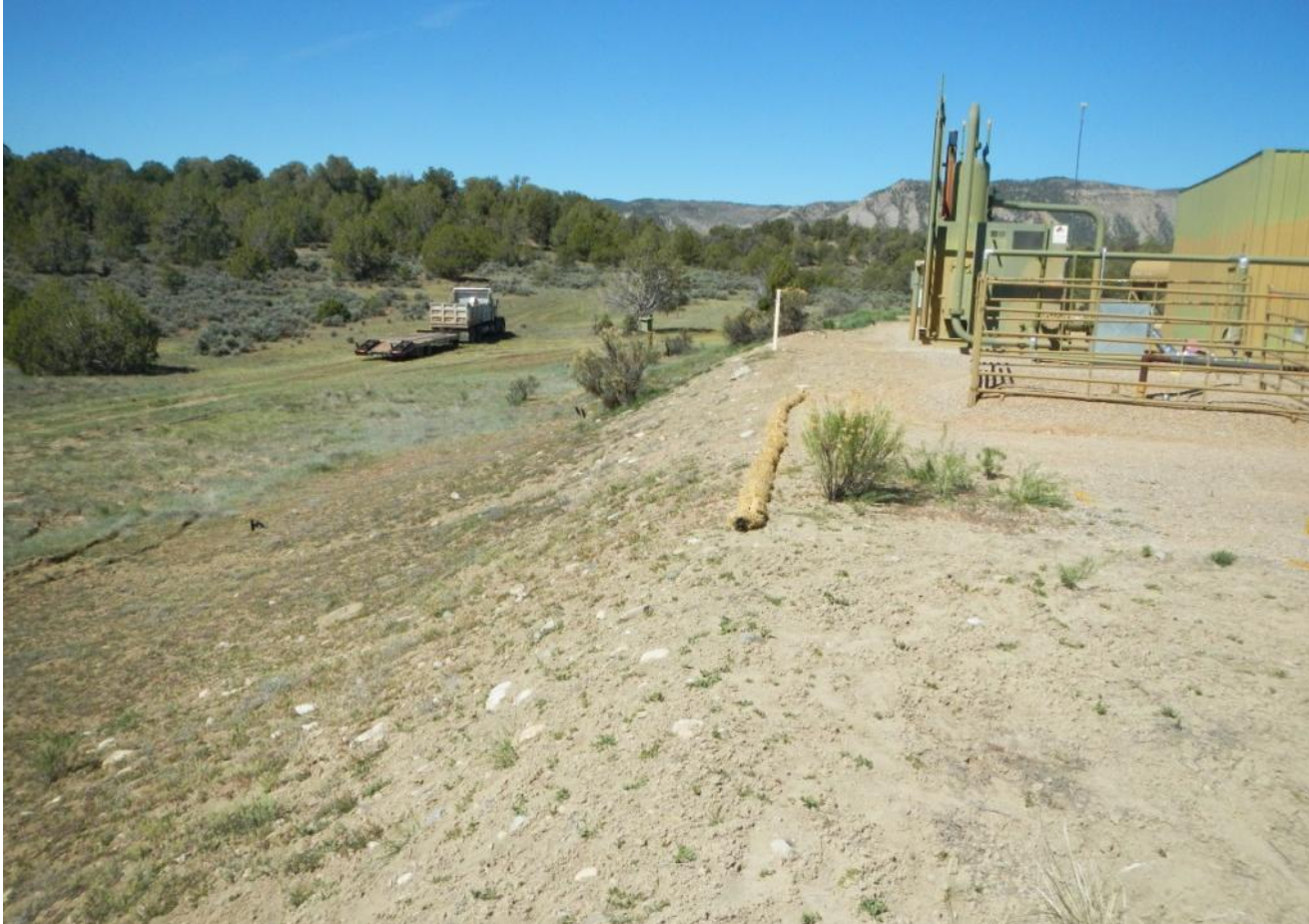
Photo 5. View of new straw wattle installation on southern edge of working area.
