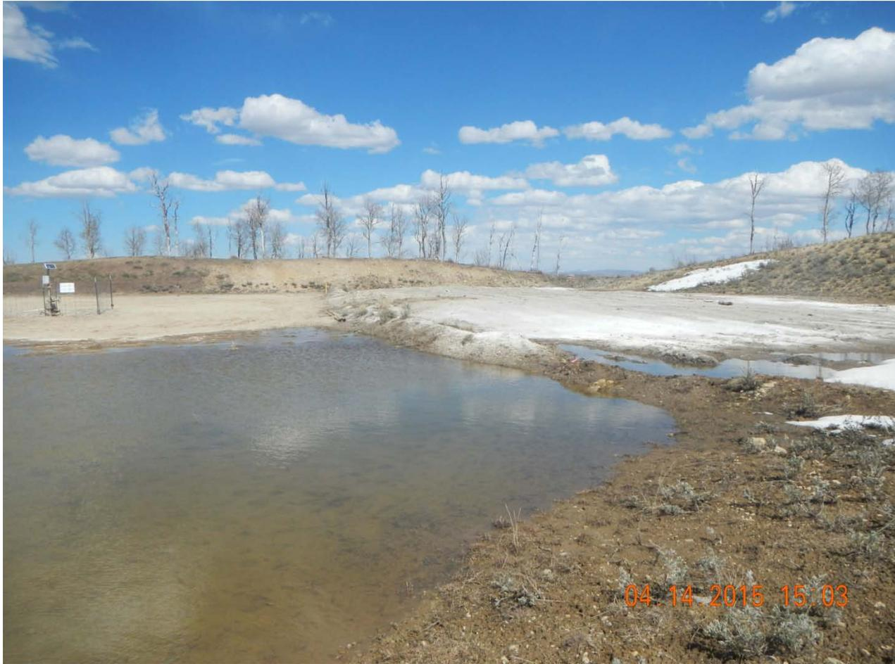
Traffic damaged berm and material piled on berm. Snow melting into land farm berm.
