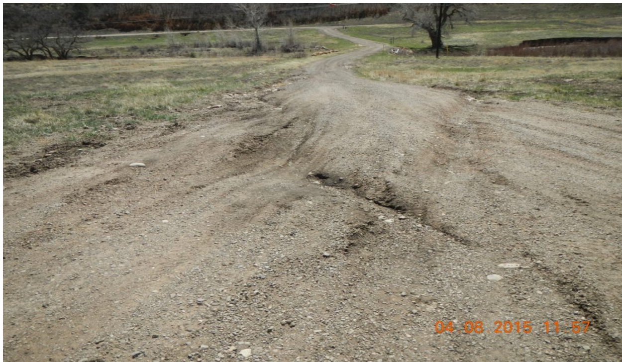
photo 3: Facing southeast towards the access road. Erosion channels developed across the access road.
