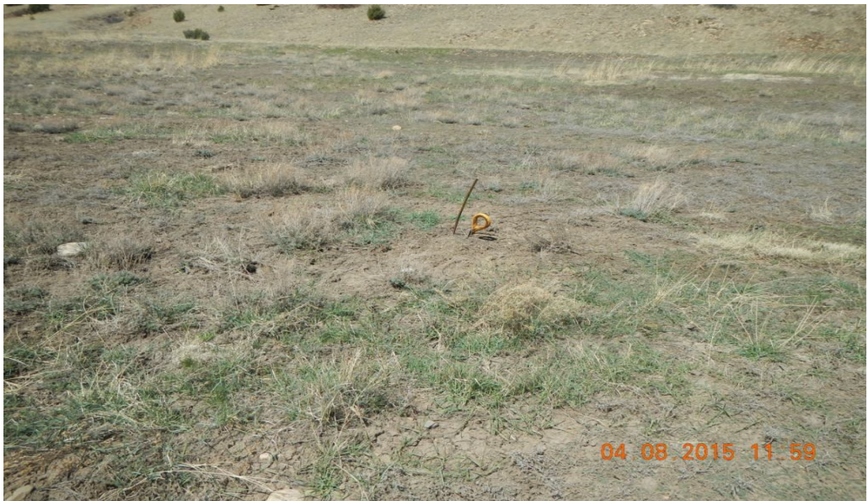
photo 6: Guy line anchor is not properly marked.
