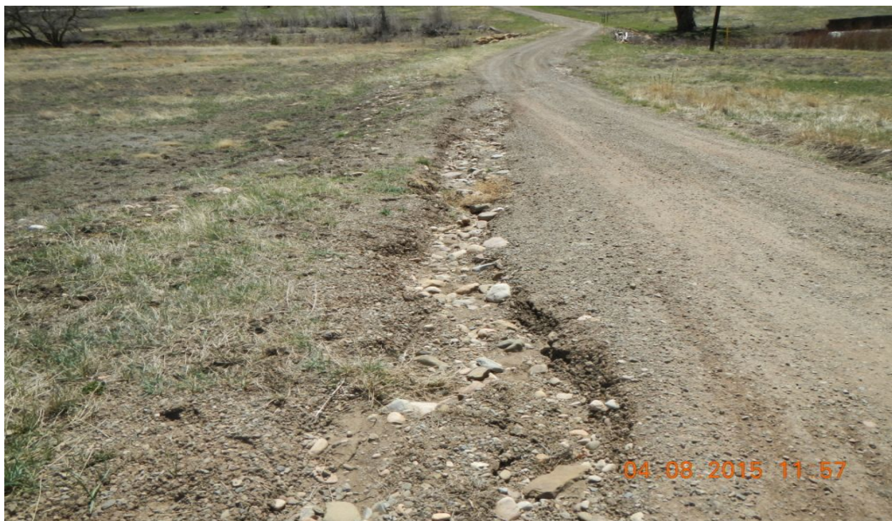
photo 4: Erosion channel along the access road.
