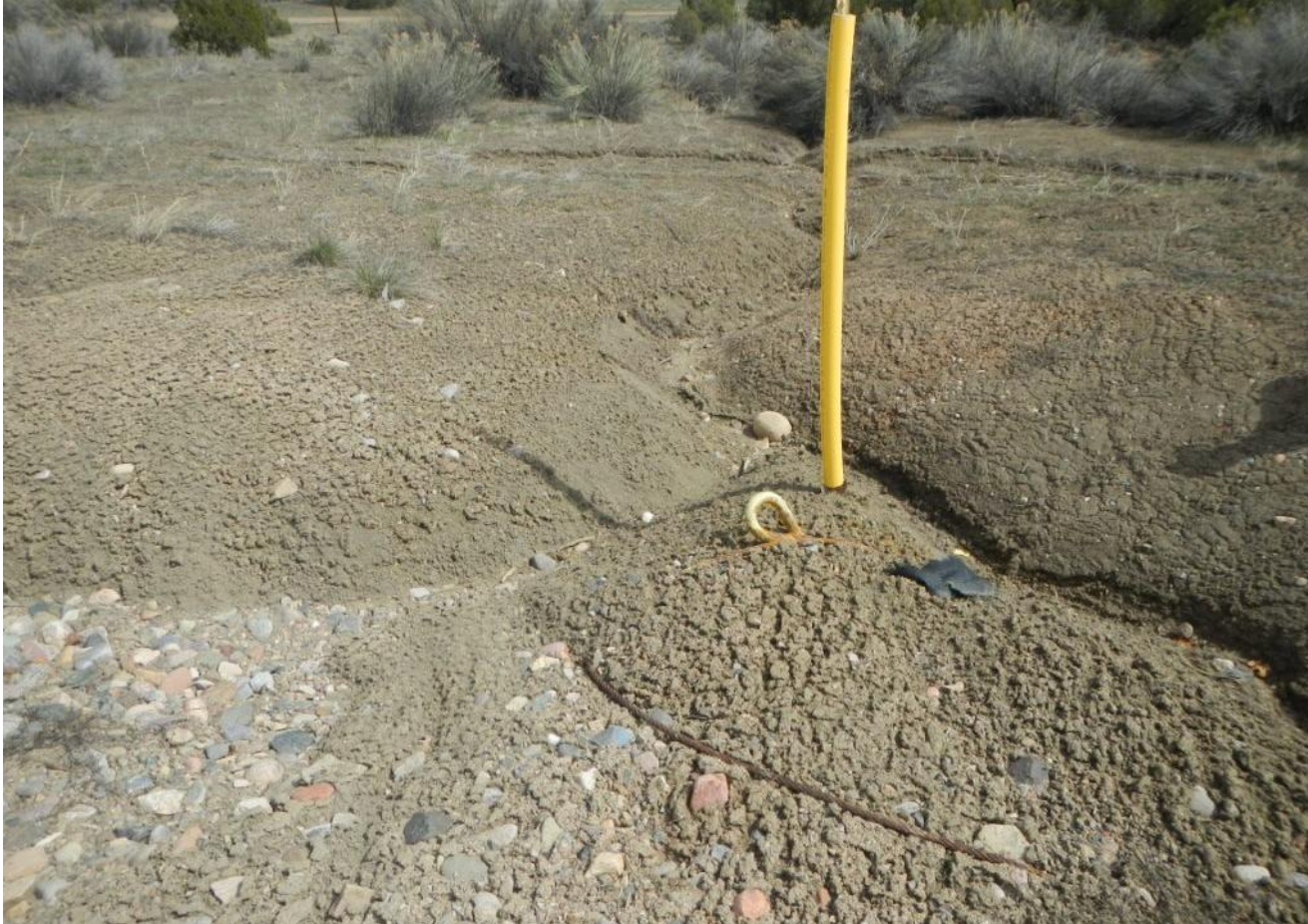
Photo 7. View of erosional channels forming along the eastern edge of the well pad. Rig cable and debris can also be seen adjacent to guy line anchor.
