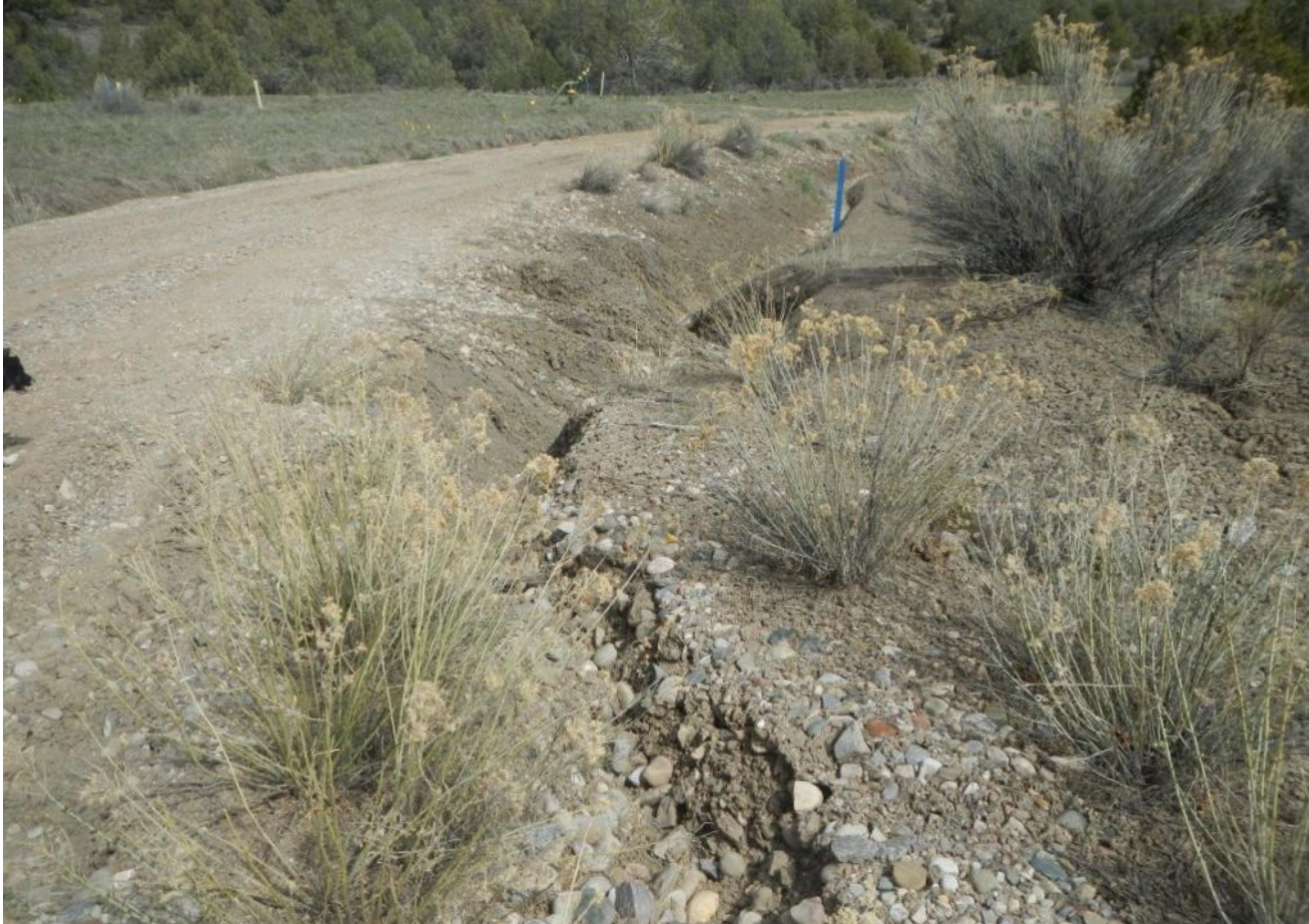
Photo 2. View of erosional channel along the southern edge of the access road.
