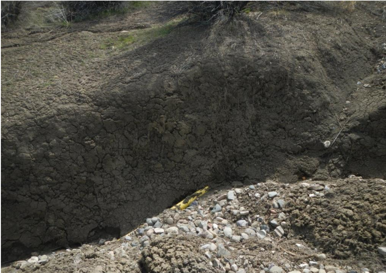
Photo 4. View of exposed pipe within the erosional channel on the southern edge of the access road.
