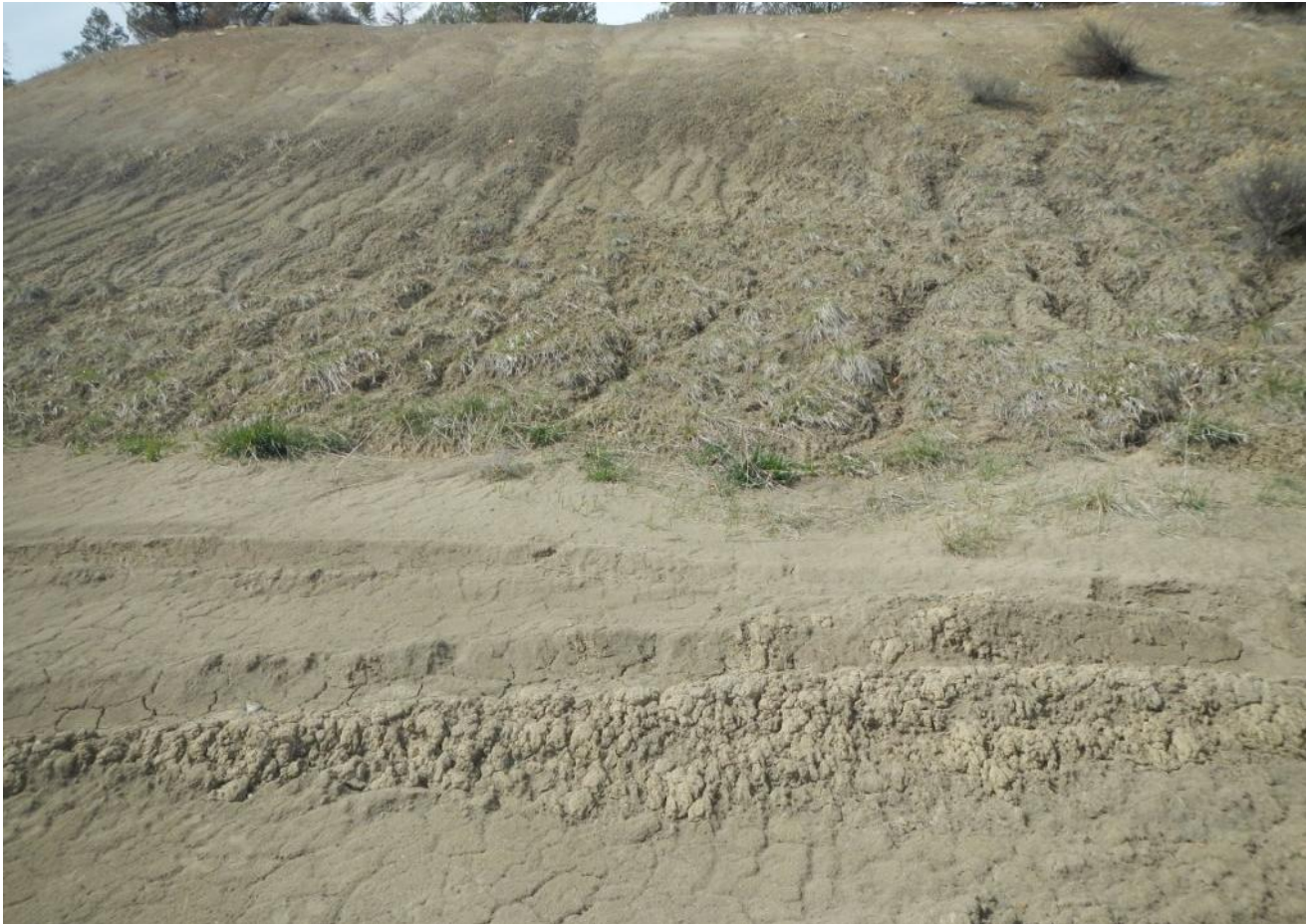
Photo 5. View of sediment deposition (bottom) and stormwater erosion (top) occurring on the well pad cut slope.
