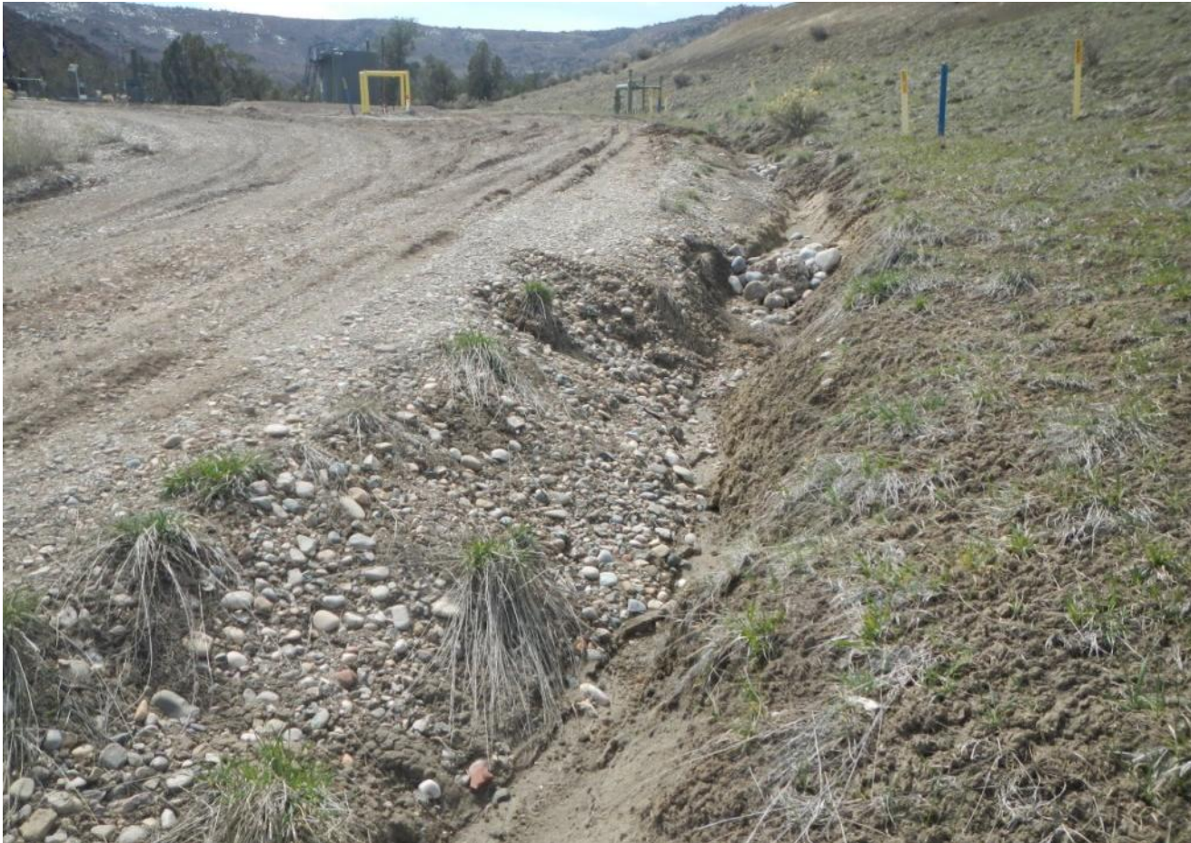
Photo 3. View of erosional channel along the northern edge of the access road.
