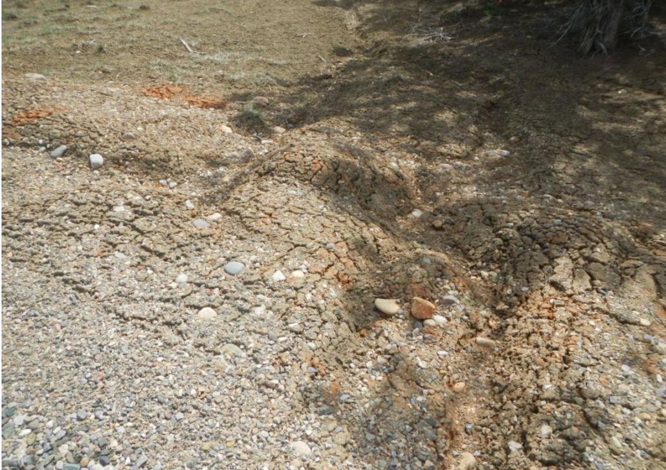
Photo 6. View of erosional channels forming along the southwestern edge of the well pad.
