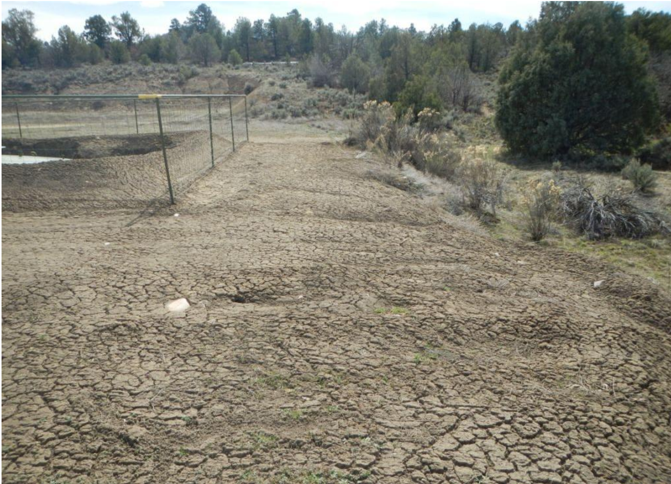
Photo 5. View of western edge of well pad where it appears stormwater flows over the edge, eroding the well pad surface.
