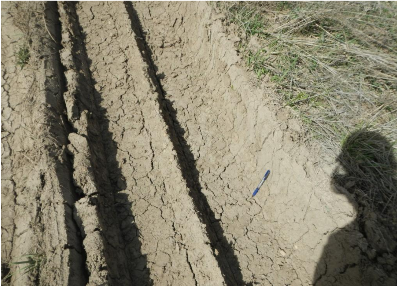
Photo 4. View of ruts approximately 12 inches deep within access road.
