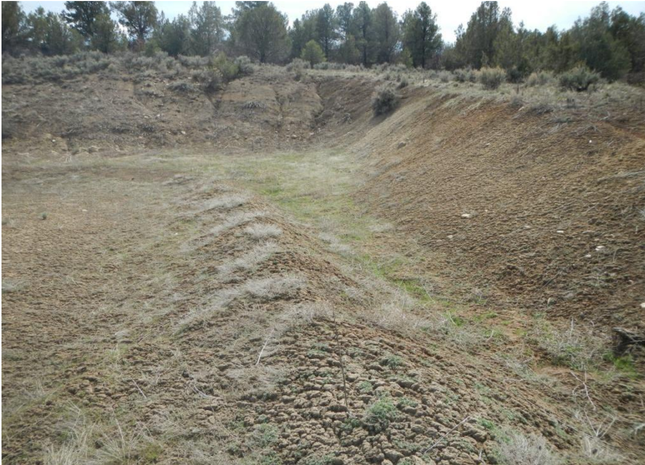
Photo 3. View of cut-slope in southwestern portion of well pad. Poor revegetation along cut-slope. Vegetation at the toe of the slope is largely cheatgrass ( Bromus tectorum ).
