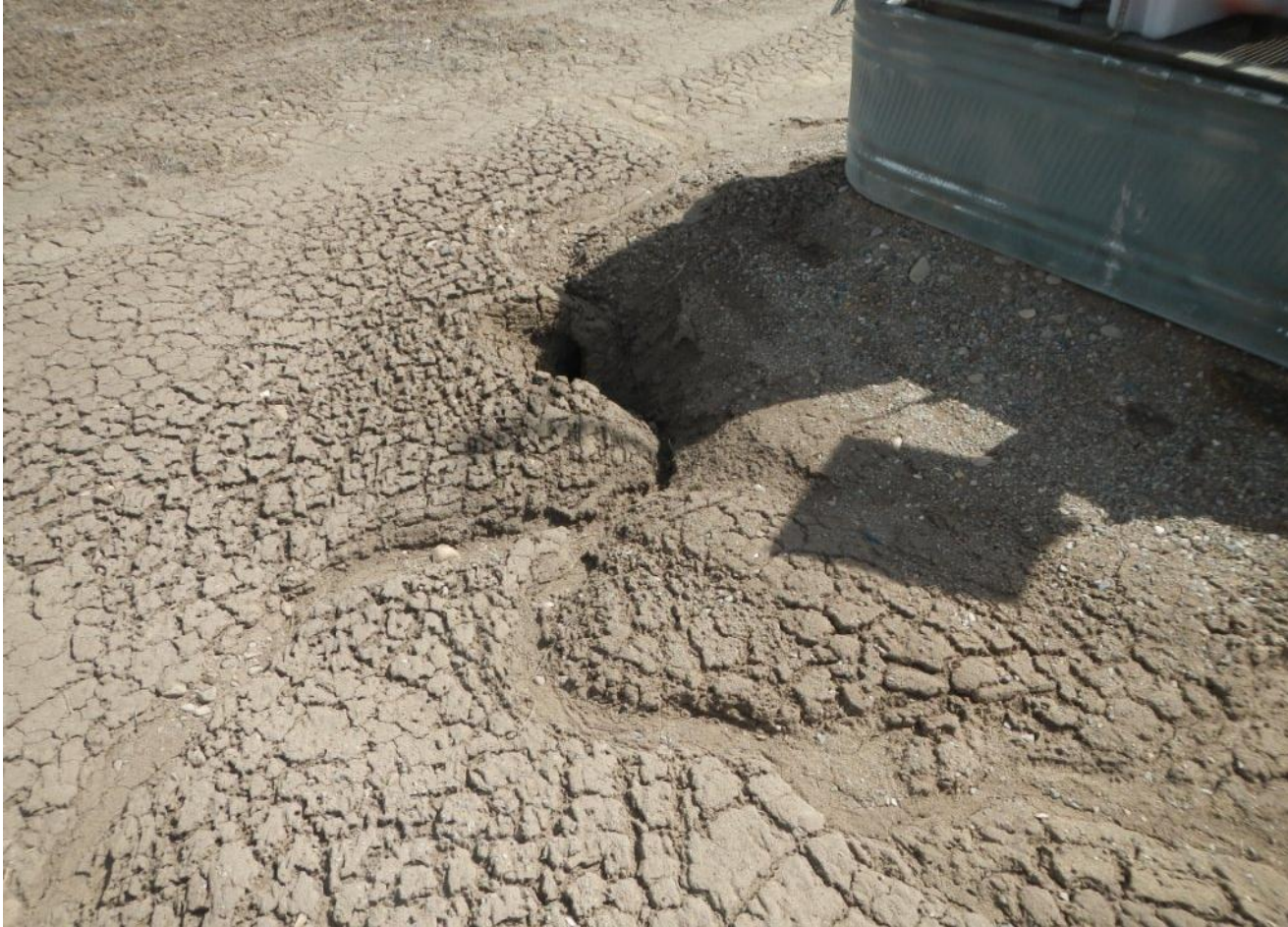
Photo 3. View of stormwater erosion channel forming within eastern portion of working surface on well pad.
