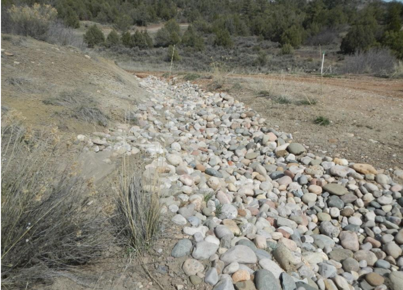
Photo 4. View of cobble-lined stormwater diversion channel along western edge of access road.
