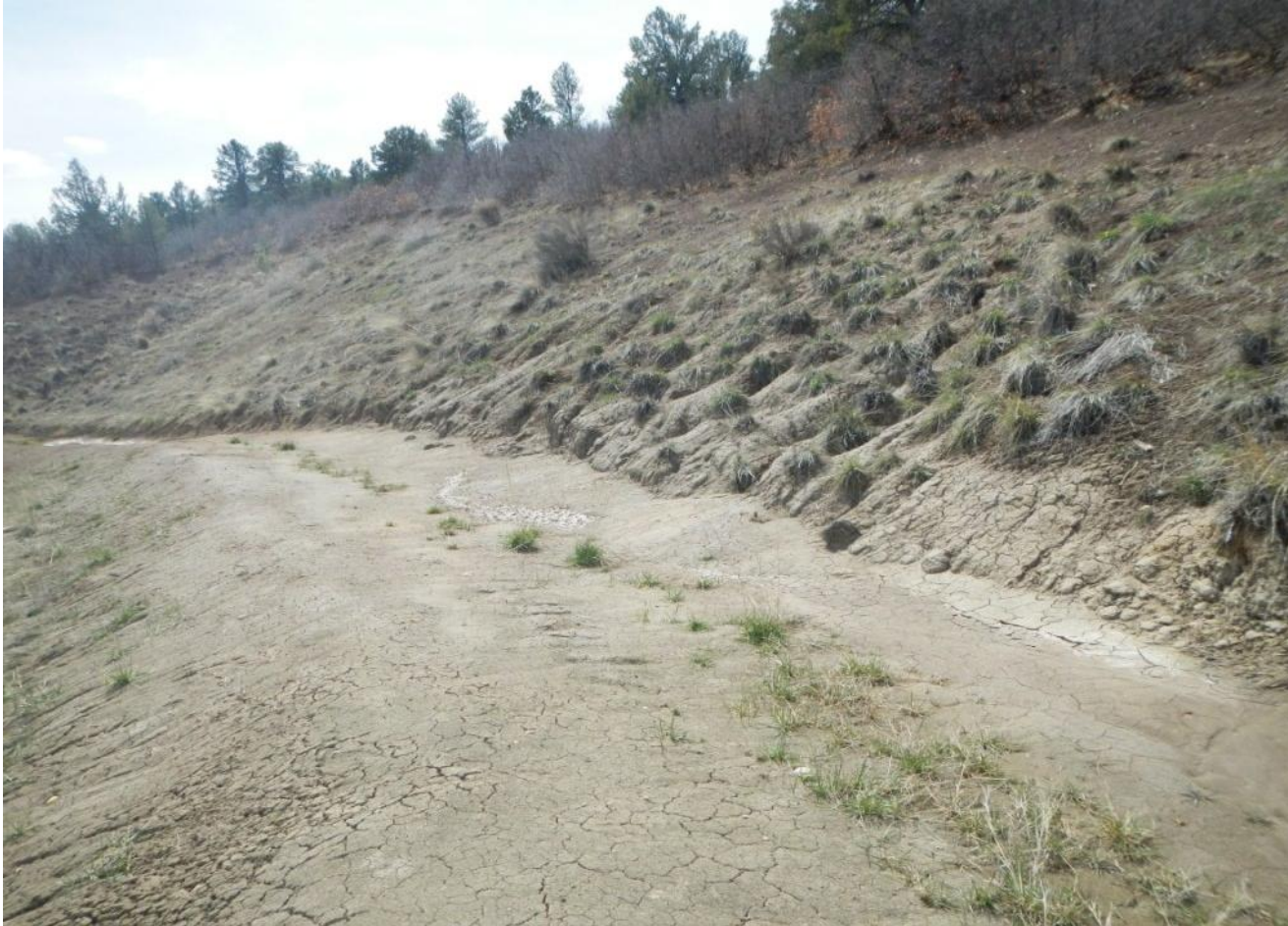
Photo 2. View of stormwater diversion in western portion of project area that is full of sediment and needs maintenance.
