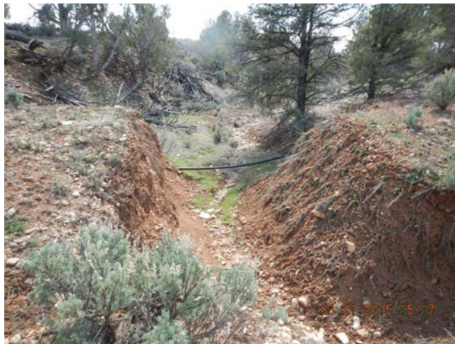
View of access road washout
