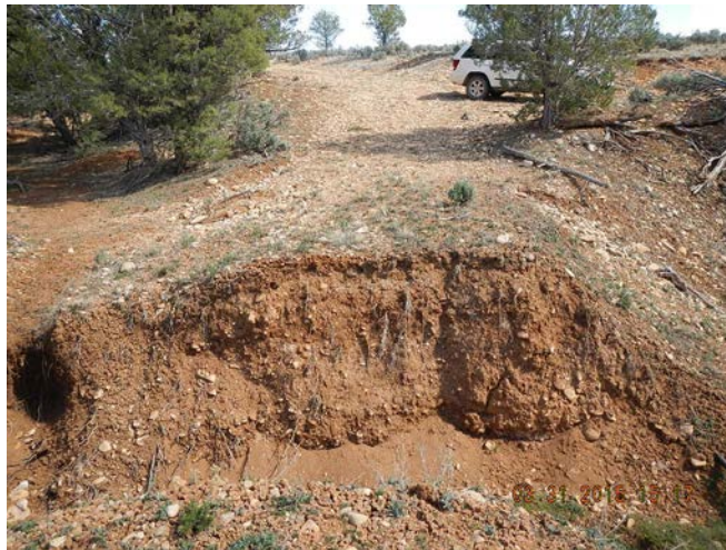
Access road washed out at drainage crossing
