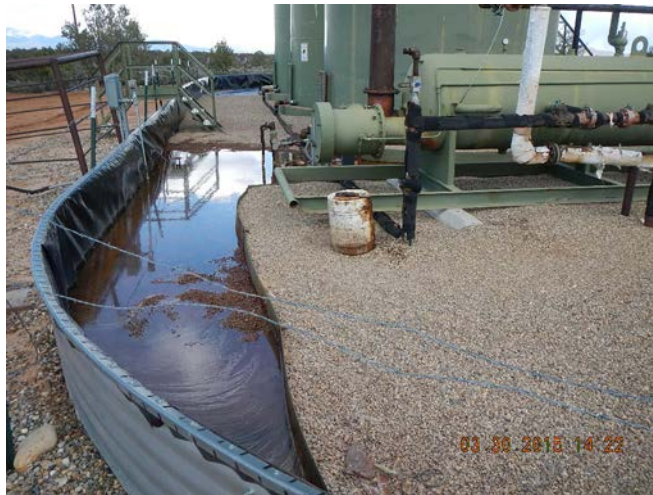
Stormwater accumulation in berm area
