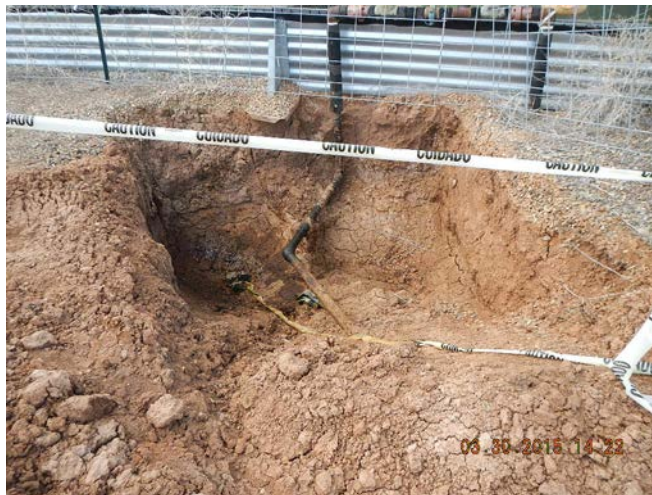
Flowline leak in excavation
