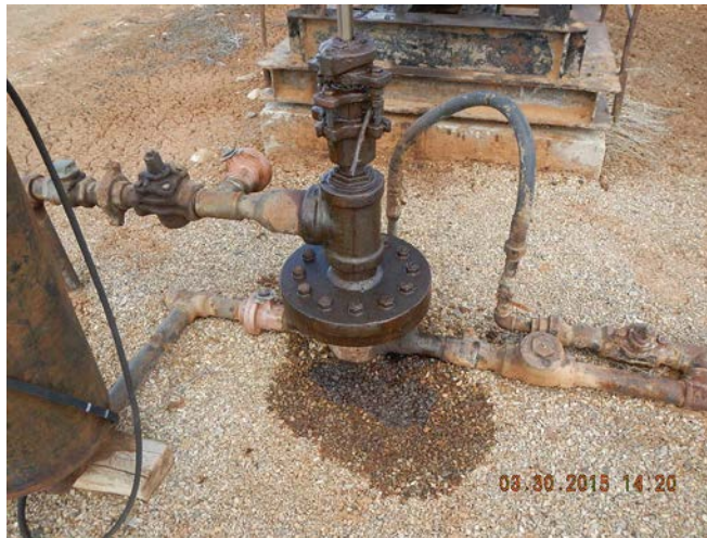
Leak at wellhead
