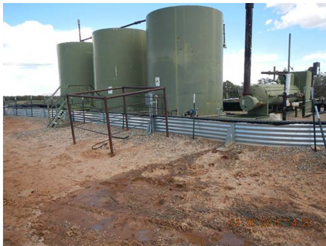
Stormwater leak onto well pad from berm area
