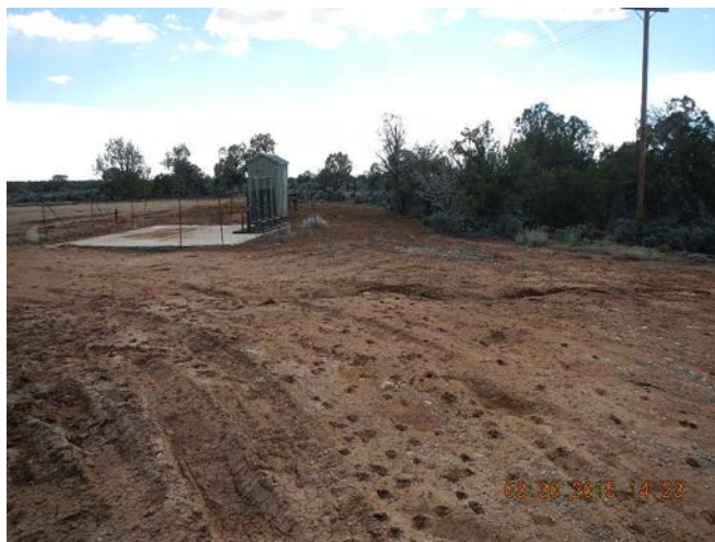
Stormwater erosion channel on well pad
