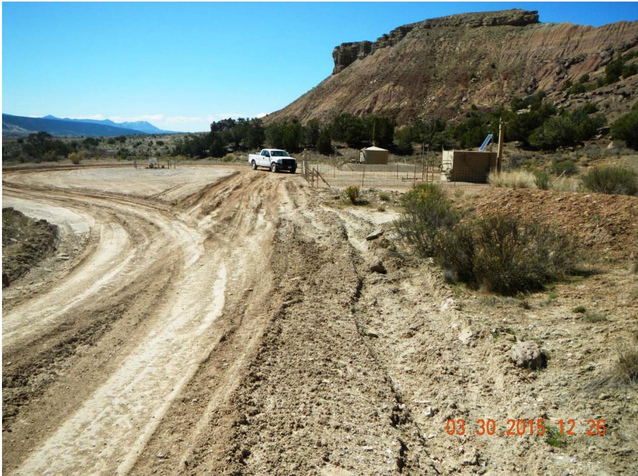
Outlet side of check dam is washed away.
