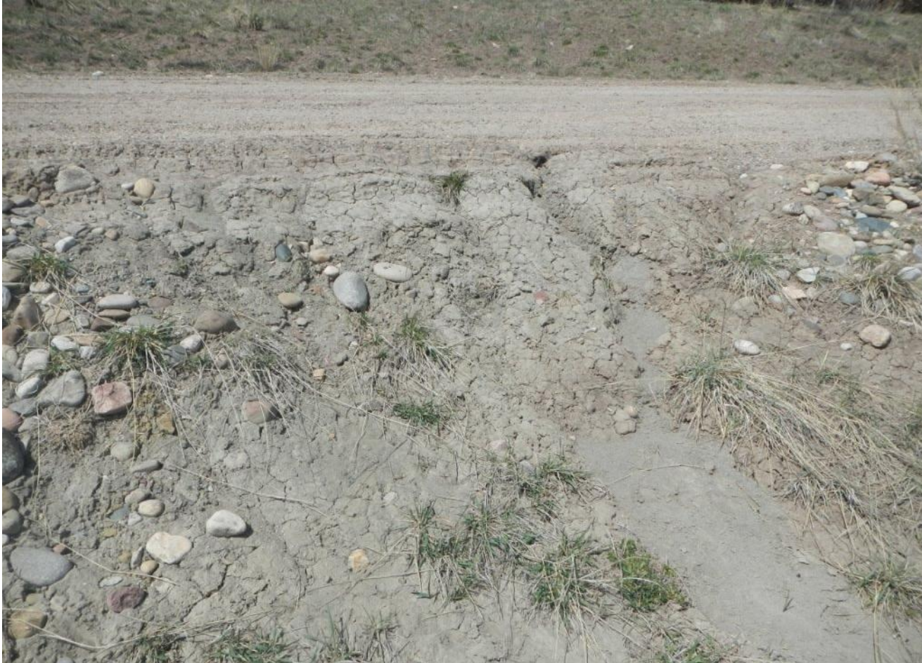
Photo 3. View of rill erosion on shoulder of access road.
