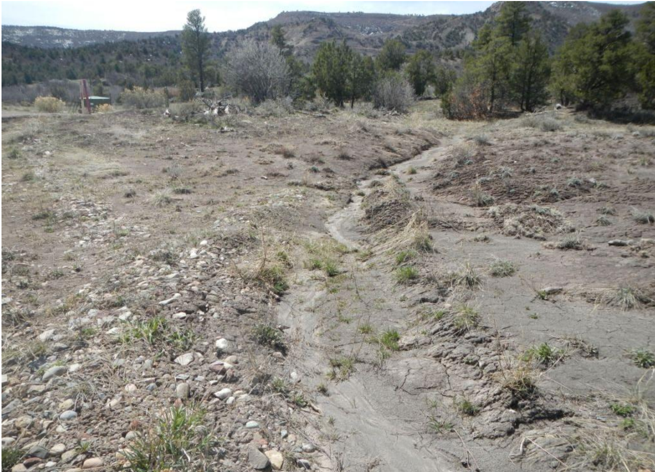
Photo 4. View of bar ditch on western side of access road. Stormwater flows along bar ditch are not sufficiently de-energized and causing erosional downcutting.
