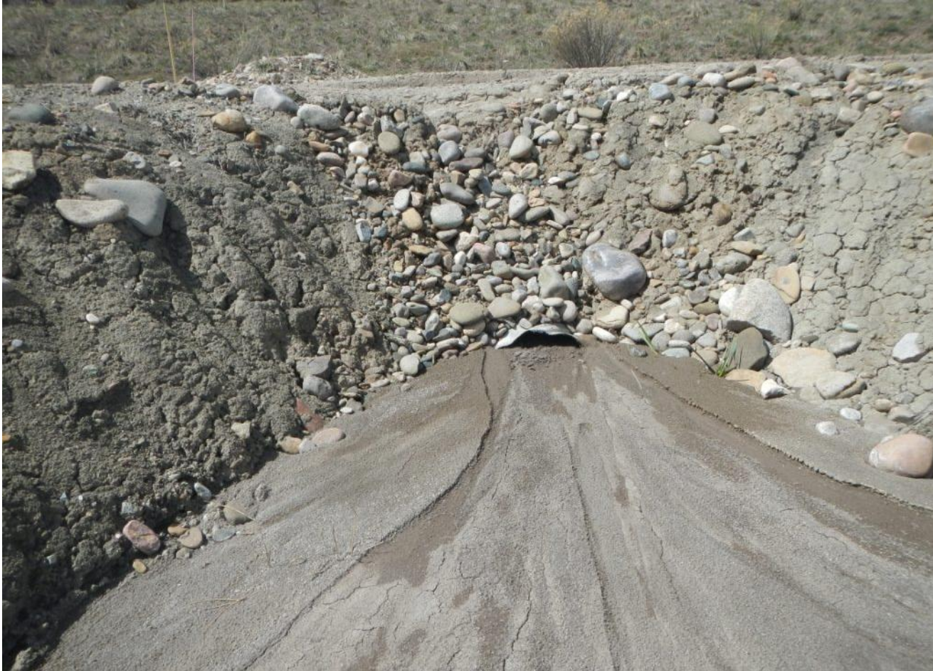
Photo 2. View of culvert outlet near entrance to well pad. Culvert is largely full of sediment.
