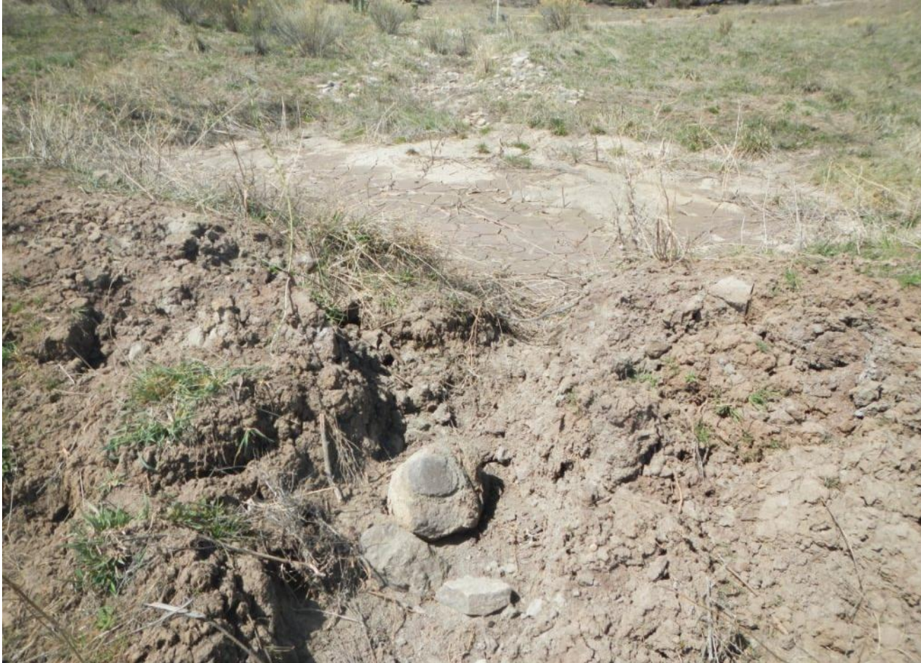
Photo 6. View of silt trap in southern portion of project area. A breach in the berm can be seen in the center of the photo.
