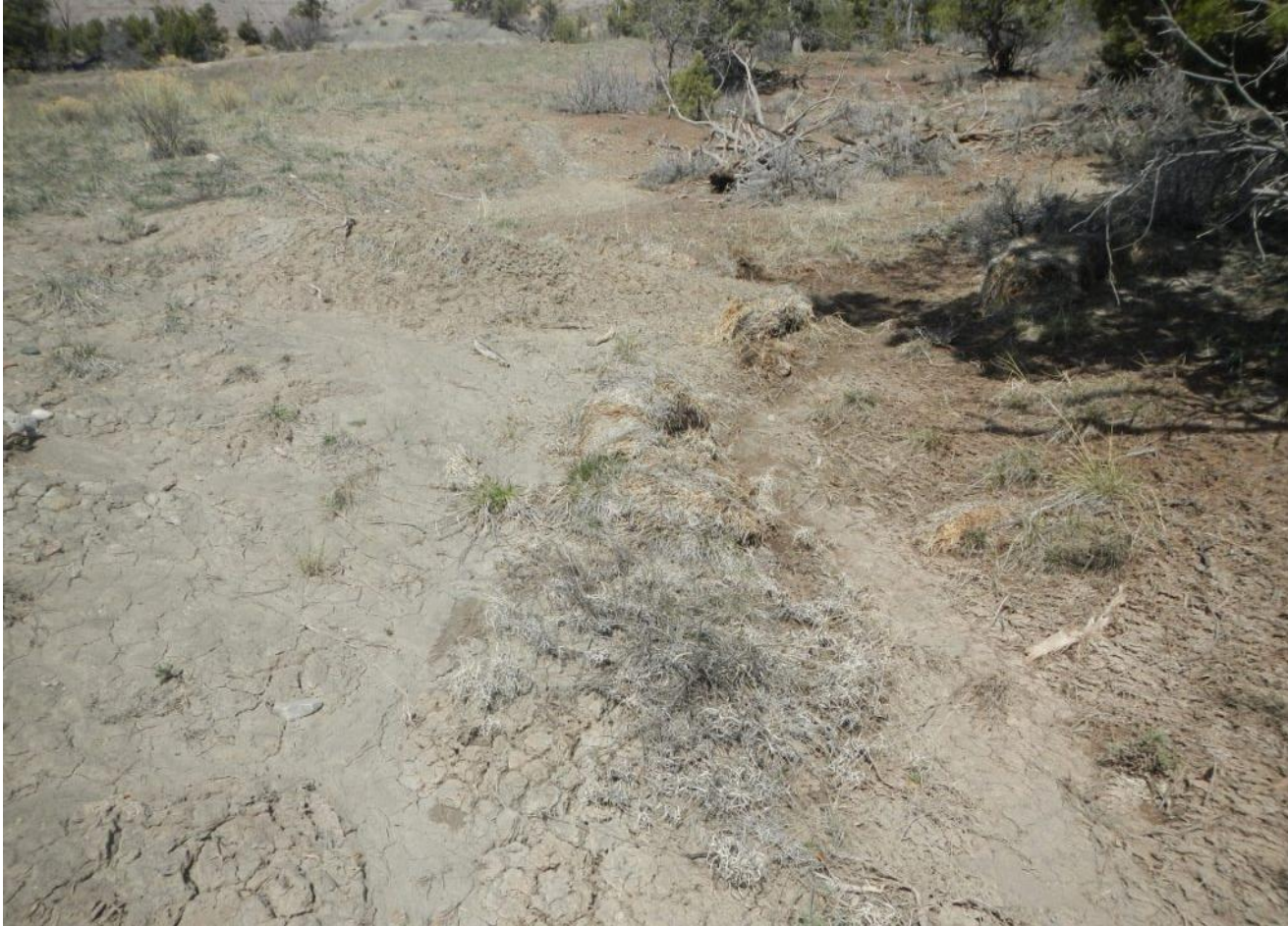
Photo 5. View of stormwater diversion along eastern edge of project area facing northward. A deteriorated silt trap berm and deteriorated straw wattles can be observed.
