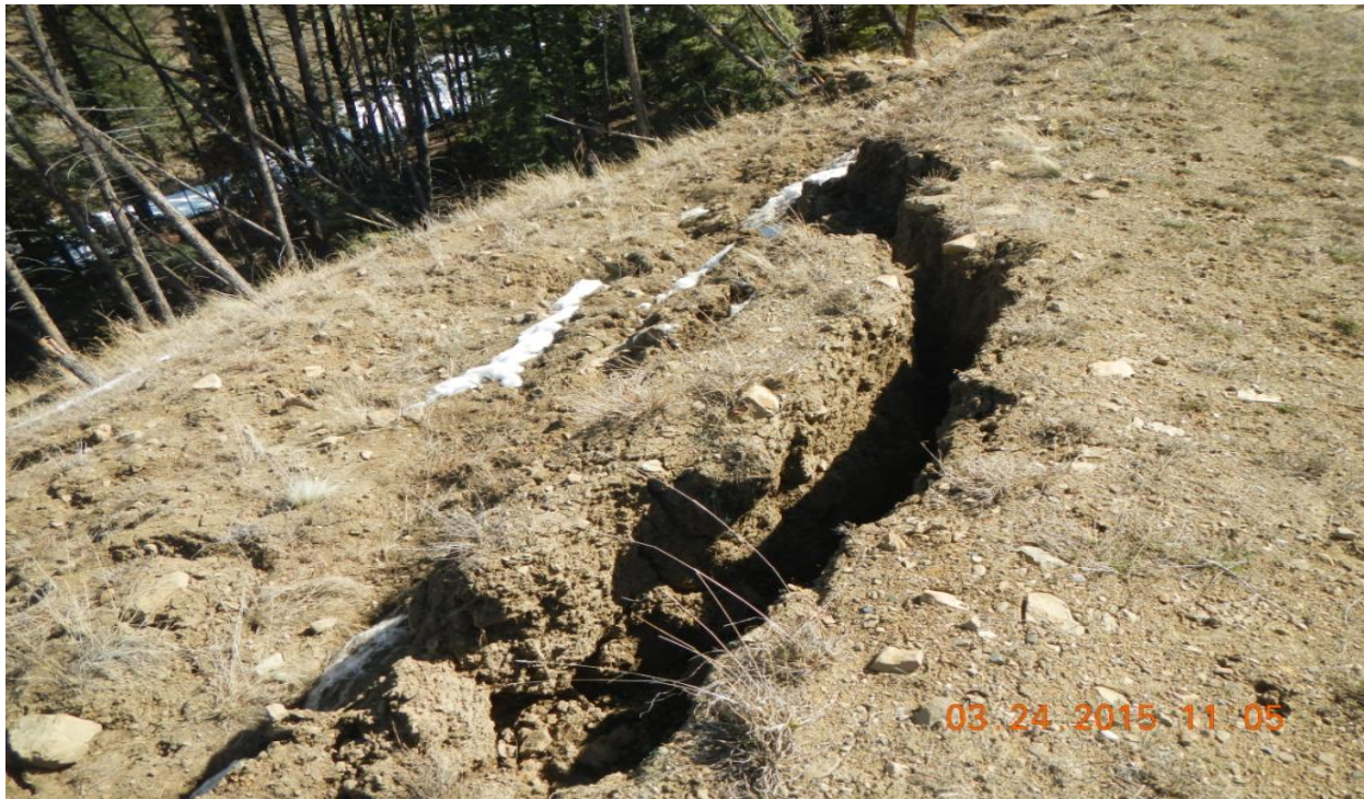
photo 7: Material sloughing off the northeast corner of the location.
