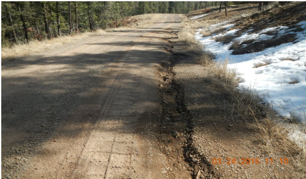
photo 8: Erosion channel along the access road.
