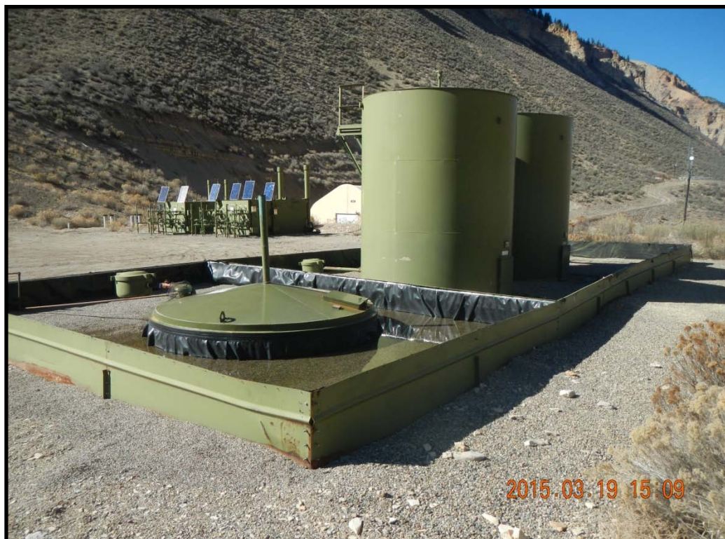
Above ground and partially buried tanks bermed and lined;
