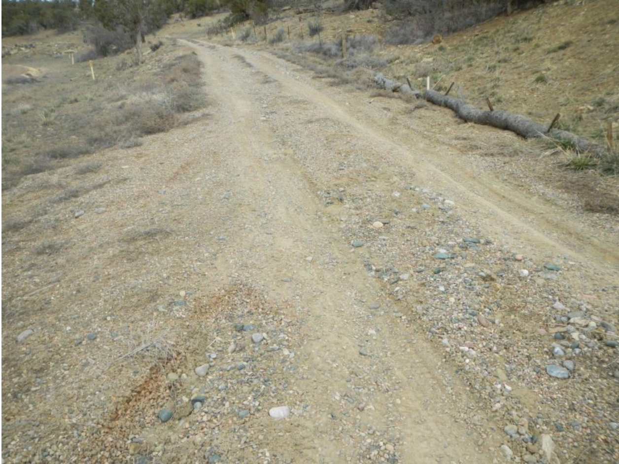
Photo 6. View of stormwater erosion along access road. A flow pattern can be seen on road and downstream (on left) where stormwater flows beneath wattles across road and down the road shoulder.
