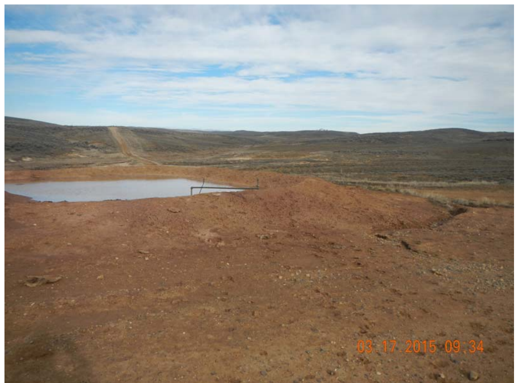
Former tank battery berm holding stormwater. Rill leaving location.
