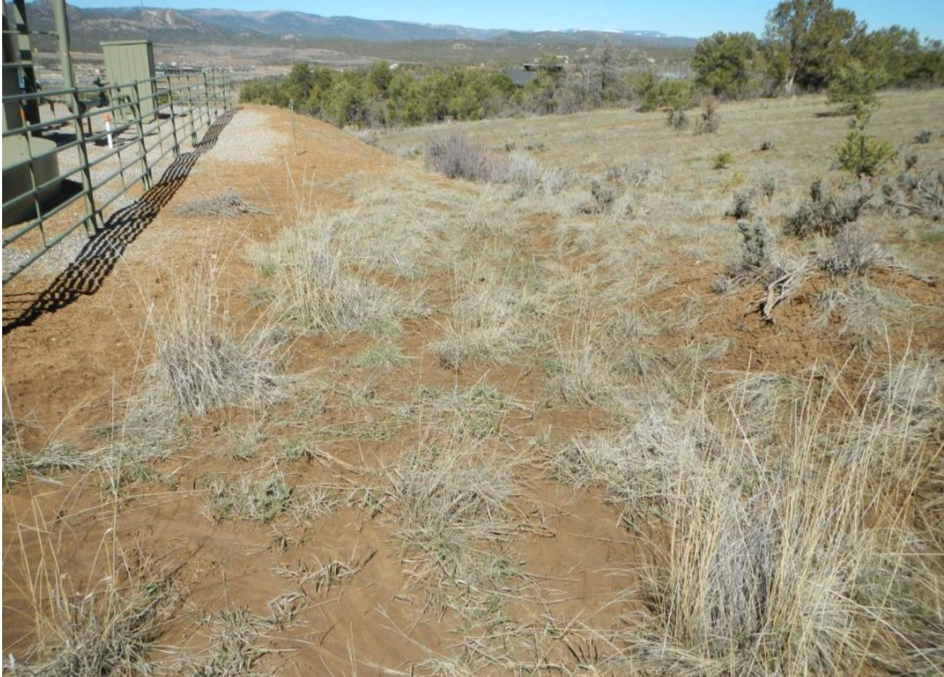
Photo 3. View of vegetated stormwater diversion channel in eastern portion of project area.
