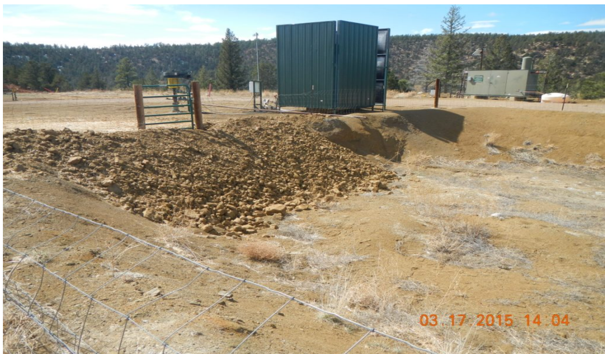
photo 8: Fence around the perimeter of the pit. Did not see a marker indicating 2ft. freeboard.
