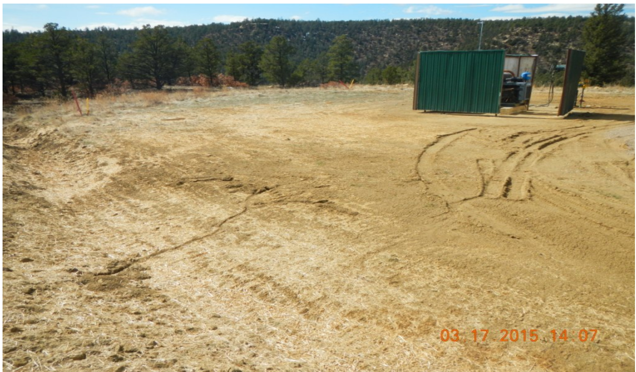
photo 6: Southeast corner of the location facing west.
