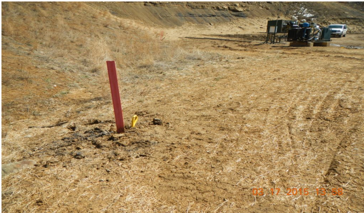
photo 4: North side of the location facing southeast.
