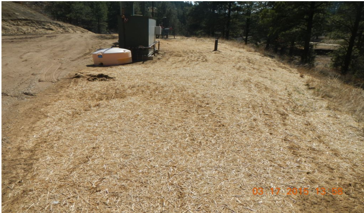
photo 3: West side of the location facing south. Area has recently been mulched.
