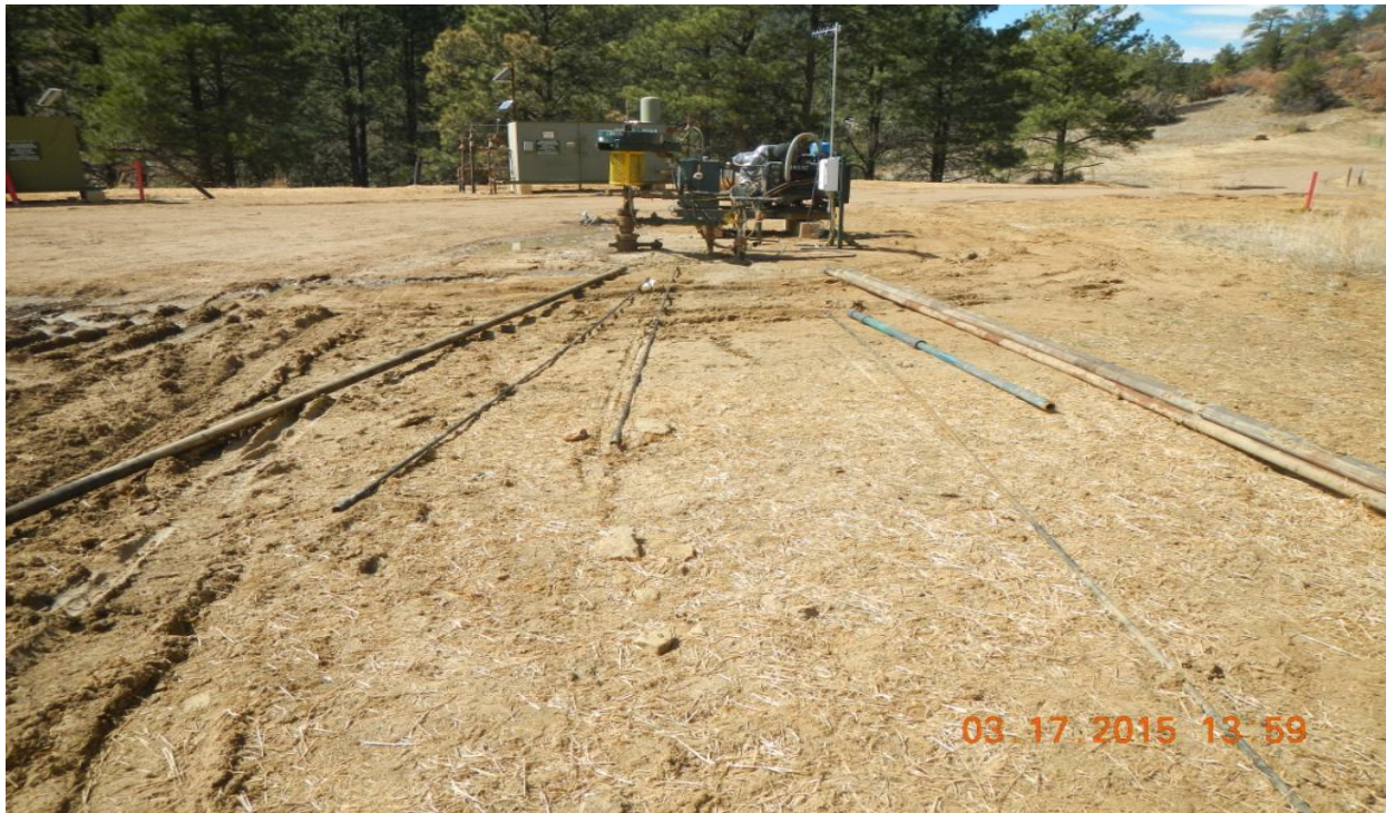
photo 5: Unused pipe was left at the location.
