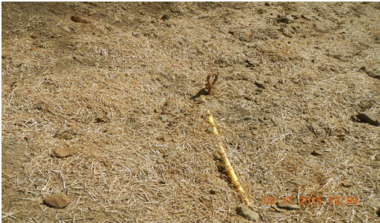
photo 6: Guy line anchor has fallen over at northeast corner of the location.
