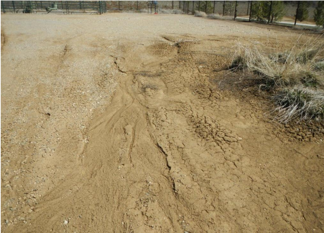
Photo 4. View of stormwater erosion on southwestern corner of working area of well pad.
