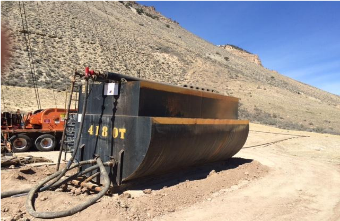
Cleaned and bermed around tank
