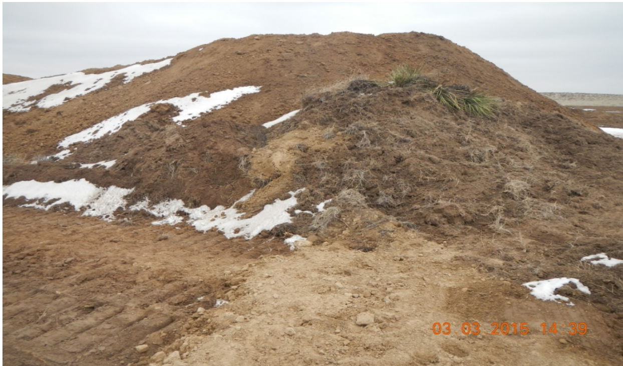
photo 13: It appears topsoil had not been properly segregated.
