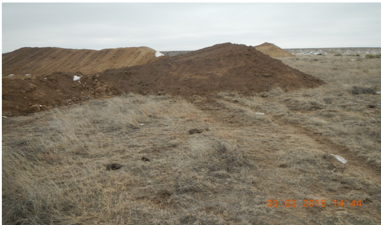
photo 11: North side of the location facing west. Dark topsoil pile separated from the drilling pit area.
