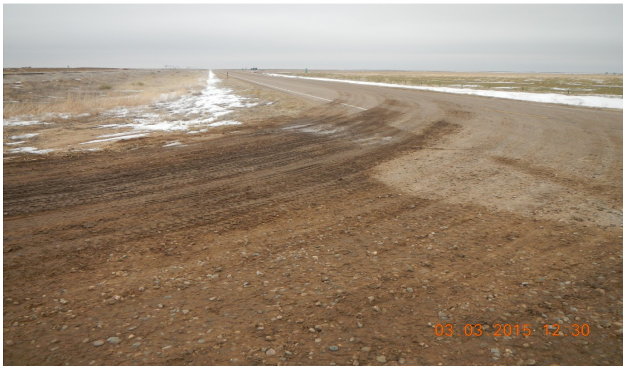
photo 18: Vehicle tracking mud onto Hwy 96 from the access road.
