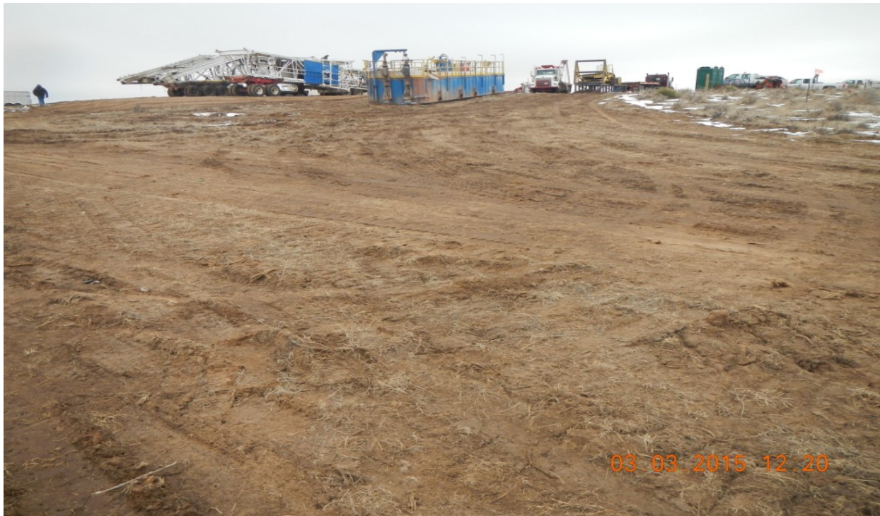
photo 5: Southwest corner of the location facing northeast.
