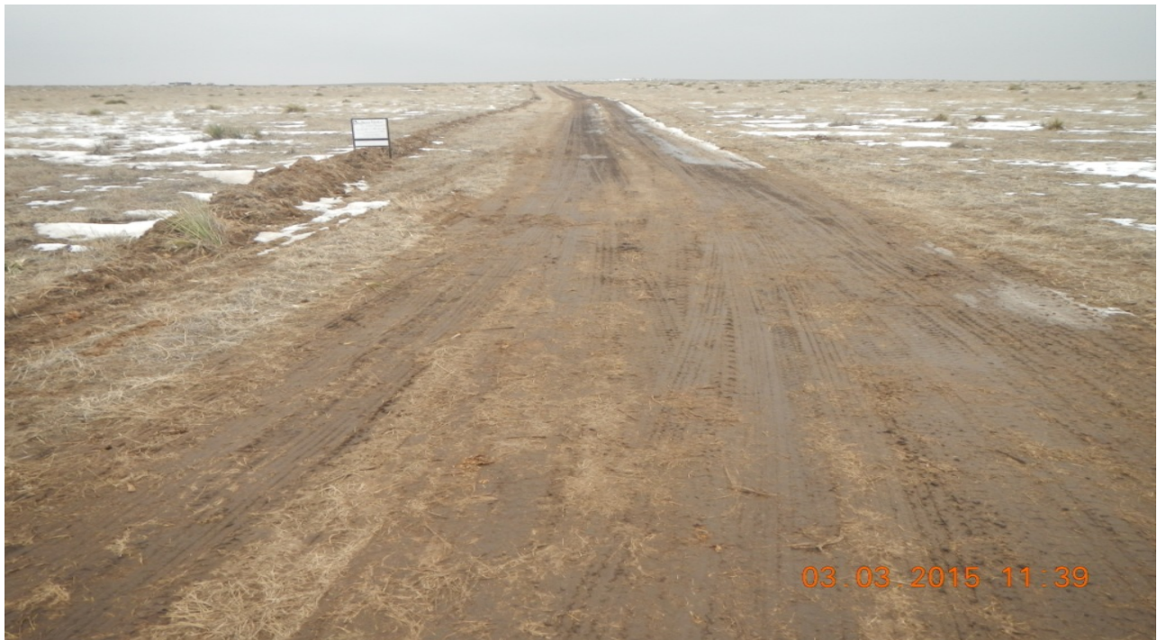
photo 2: Facing north along the access road. Topsoil was not salvaged and is being heavily compacted.
