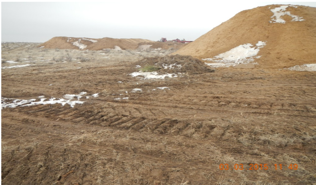
photo 12: North side of the location facing southeast.
