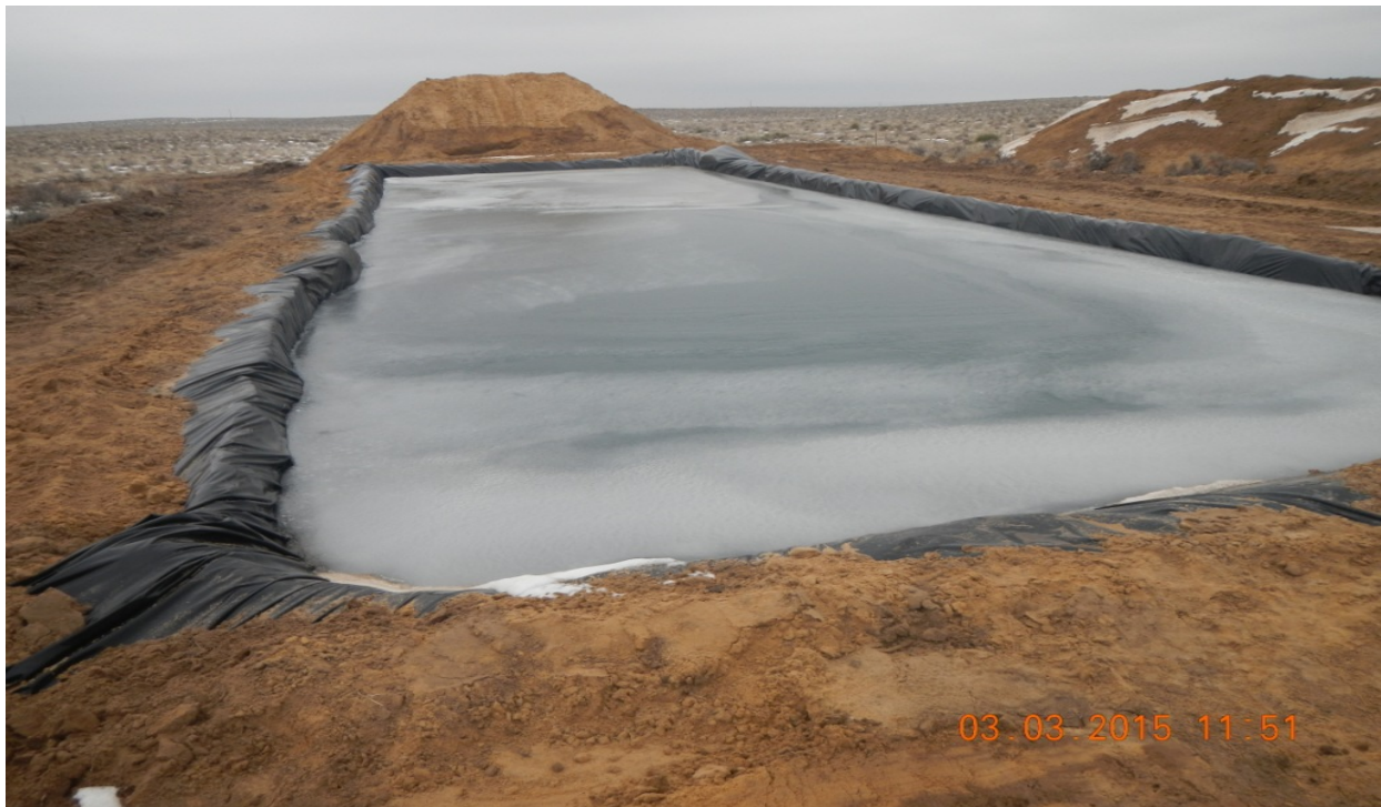
photo 14: Lined pit at the northwest corner of location does not appear to have 2ft. of freeboard.
