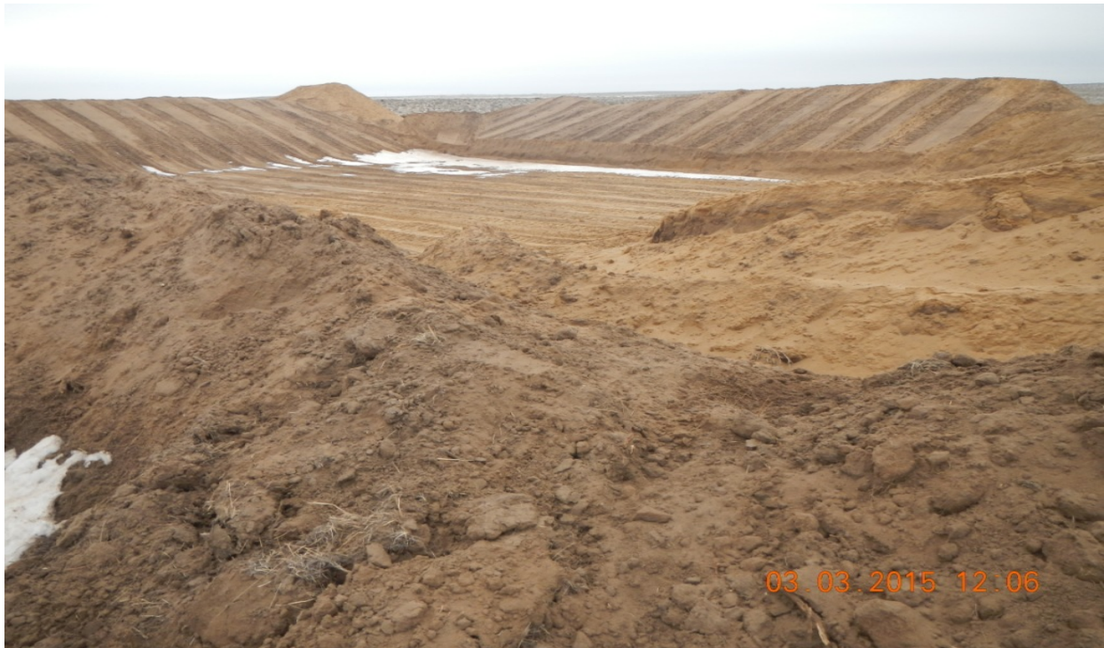
photo 11: Facing northwest towards the pit at the north side of the location.
