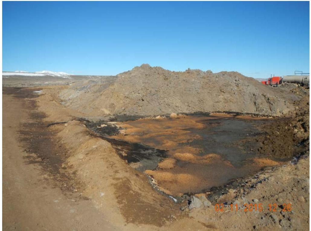
Cuttings material spilling over berm.
