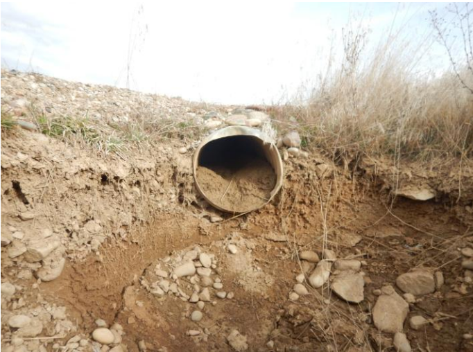
Sediment filled Culvert
