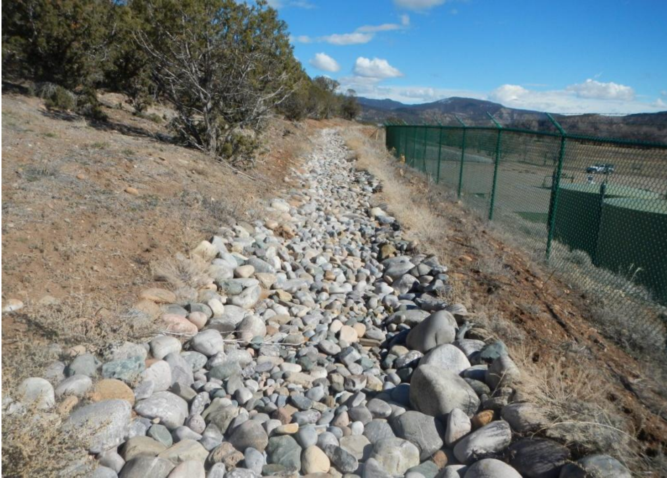
Photo 3. View of armored stormwater diversion from northwestern corner facing eastward.
