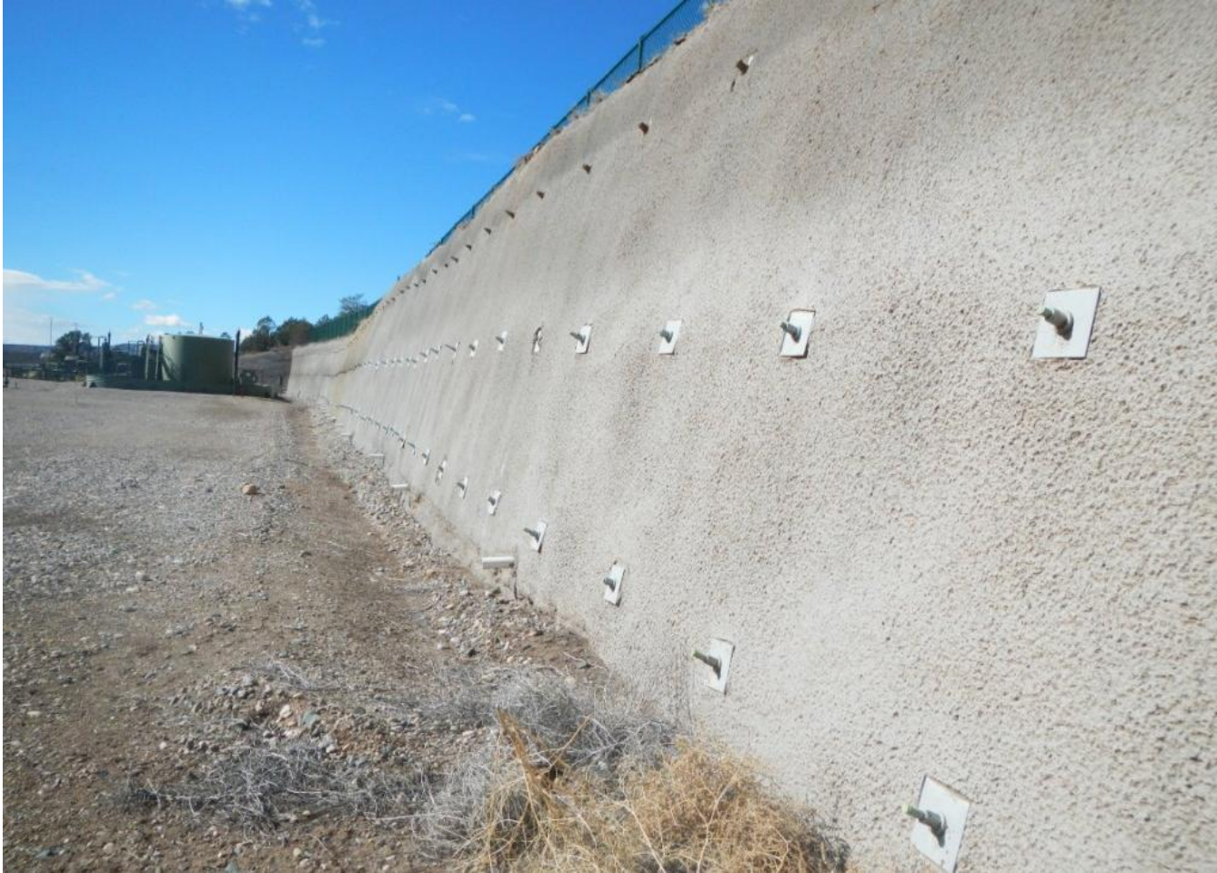
Photo 1. View of concrete stabilization of northern cut-slope.
