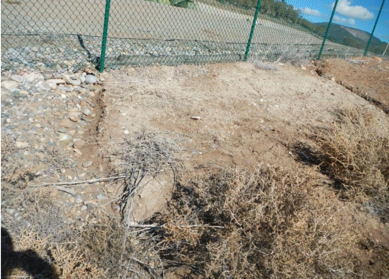
Photo 4. View of rill erosion forming in southern portion of project area. Successful revegetation of this area would provide better stabilization of these slopes.
