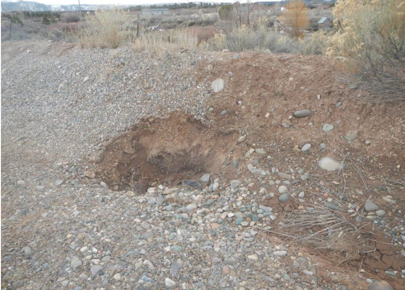
Photo 4. View of area in southern berm where it appears that stormwater flows have eroded a hole that flows through the well pad.
