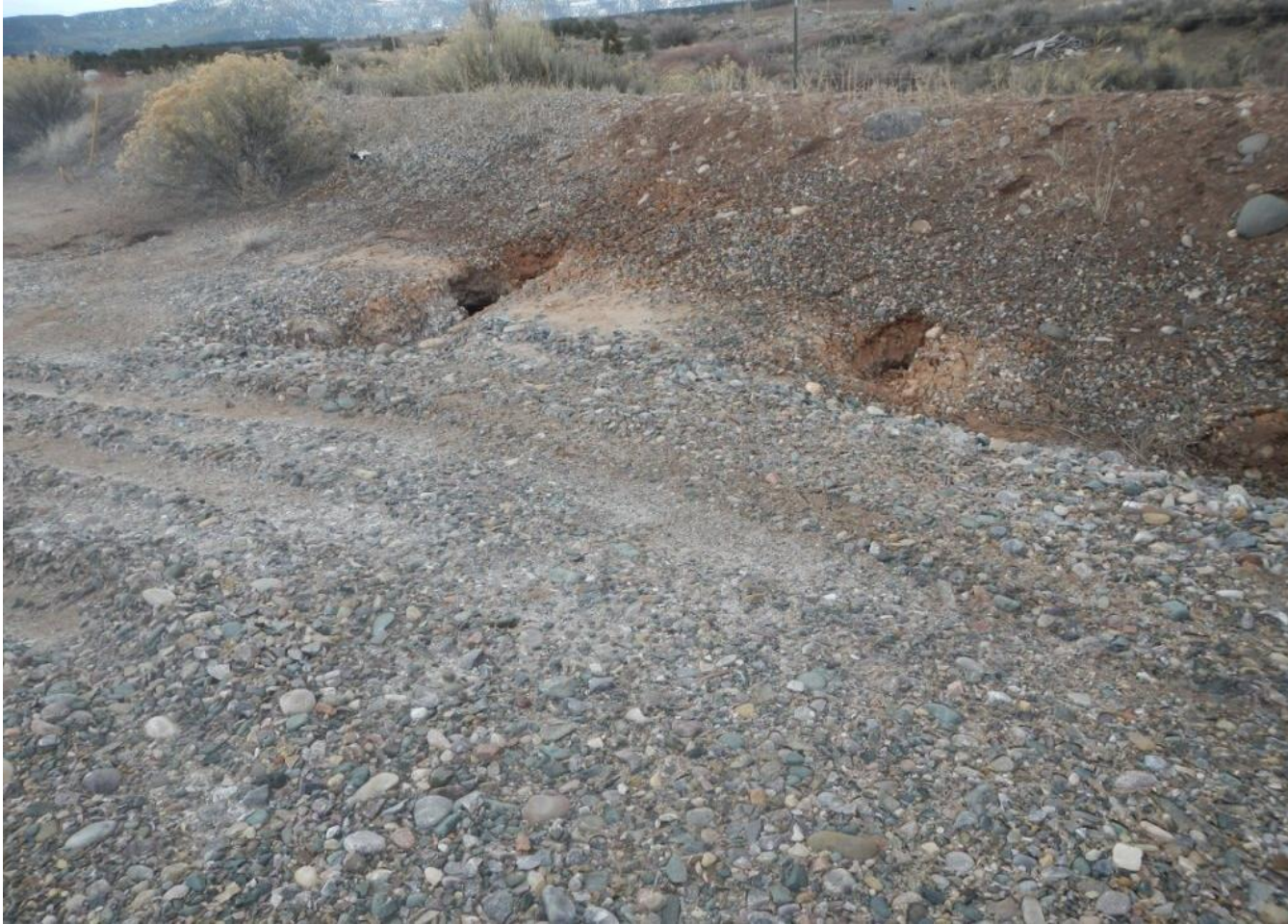
Photo 5. View of additional areas in southern berm where it appears stormwater flows have eroded through the well pad.
