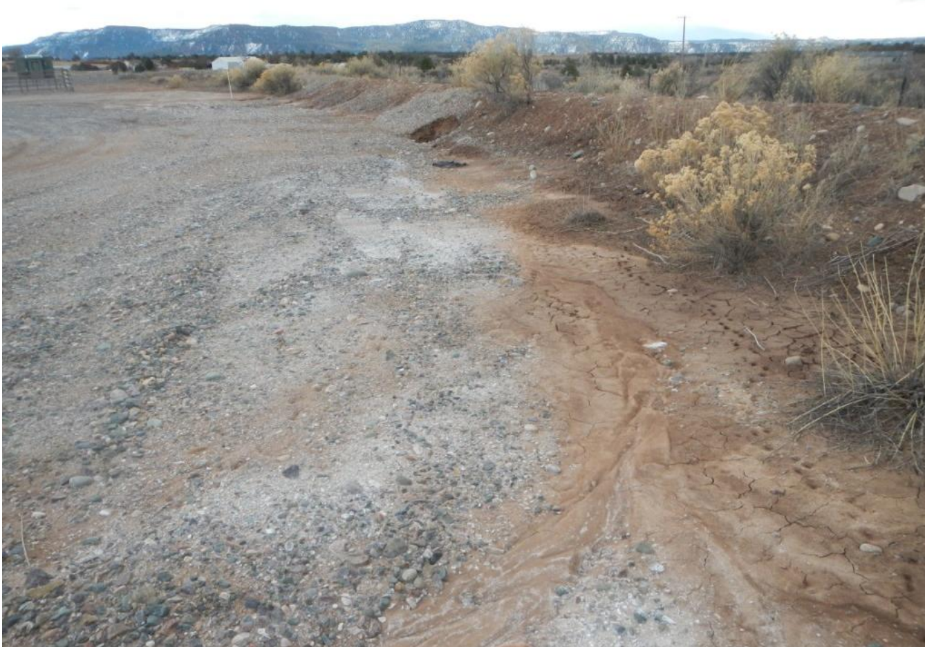
Photo 3. View of southern edge of working area from southwestern corner facing eastward. It appears that stormwater flows along southern edge and erodes through weaknesses in southern berm.
