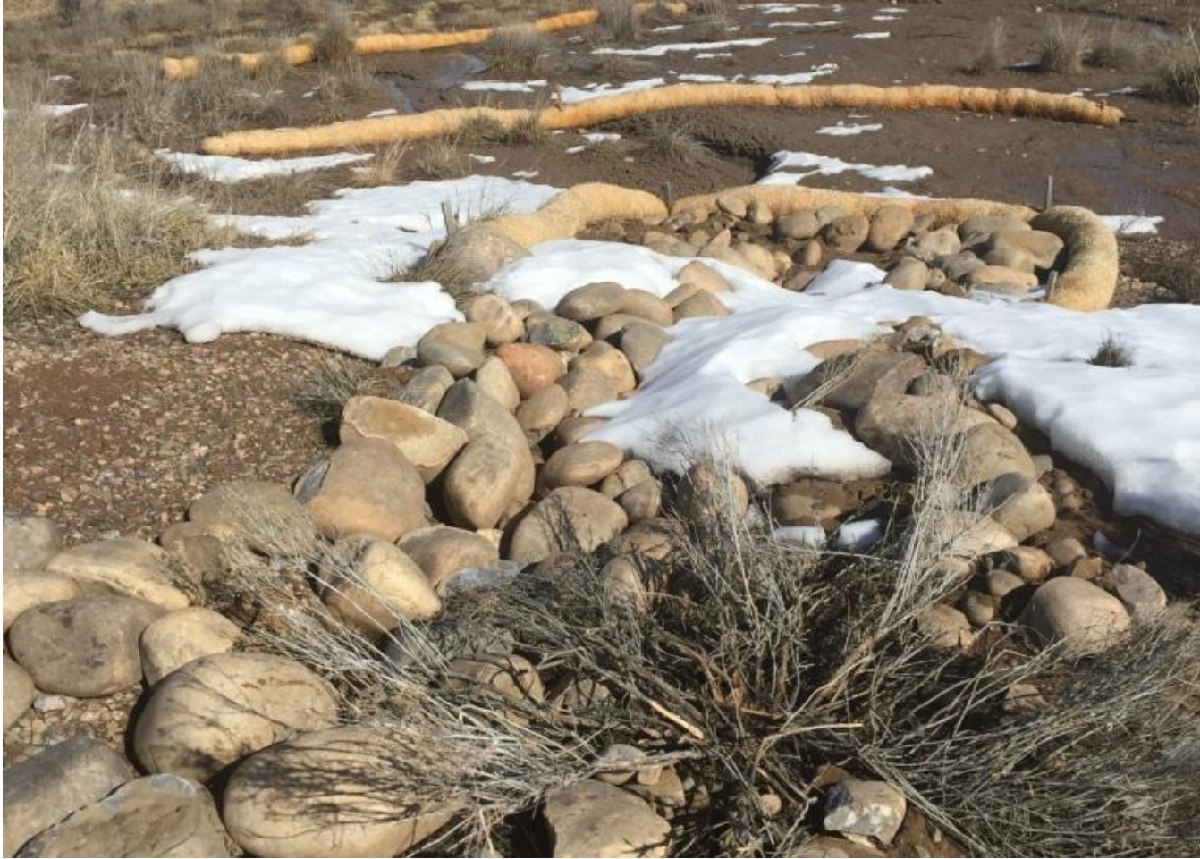
Photo 1. View of new cobble armoring and straw wattles in northeastern corner of project area.
