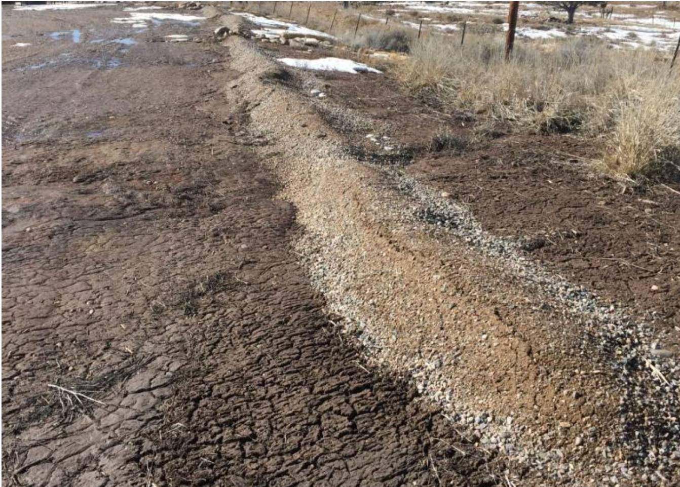
Photo 2. View of new berm along northern edge of working area.
