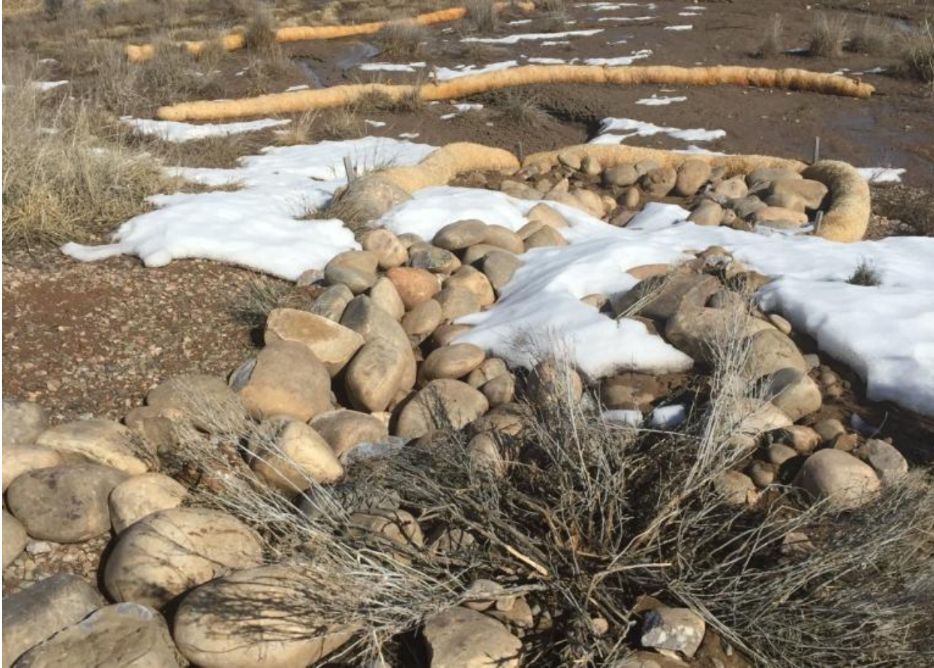
Photo 1. View of new cobble armoring and straw wattles in northeastern corner of project area.
