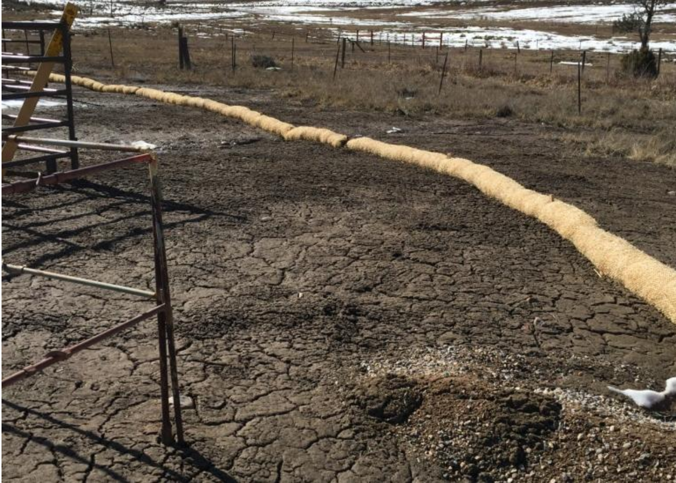
Photo 4. View of newly installed straw wattle placed along the western edge of the project area.
