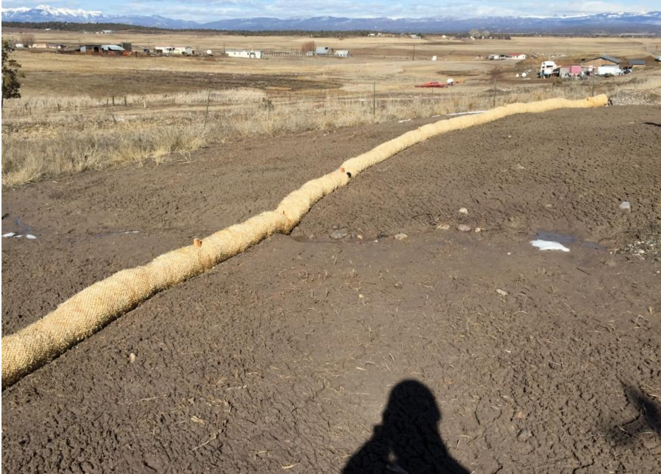
Photo 5. View of newly installed straw wattle on western edge. This will need monitoring to prevent additional sediment loss and erosion in area where erosional channels have formed.
