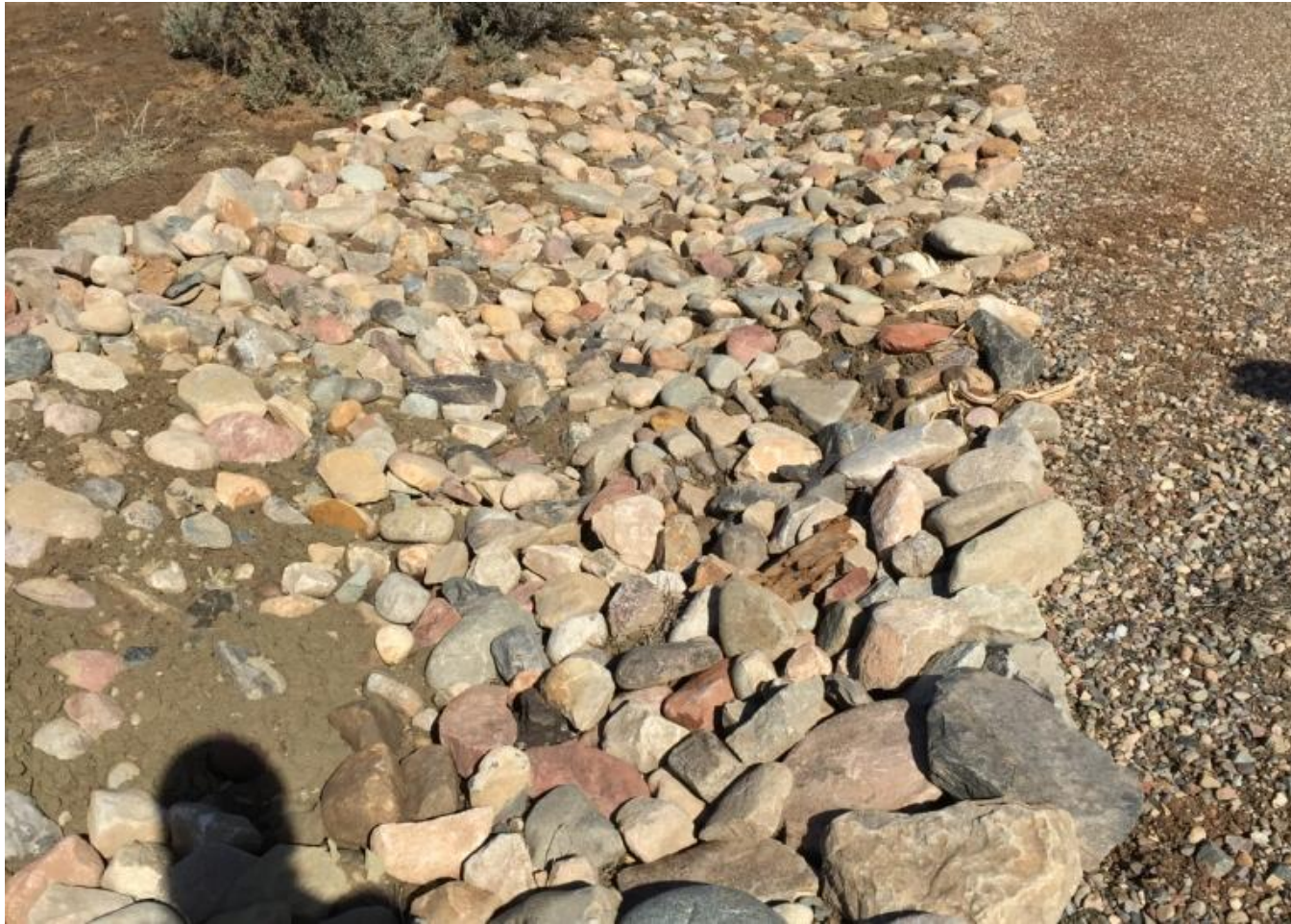
Photo 1. View of drainage diversion on the southwestern corner of project area.
