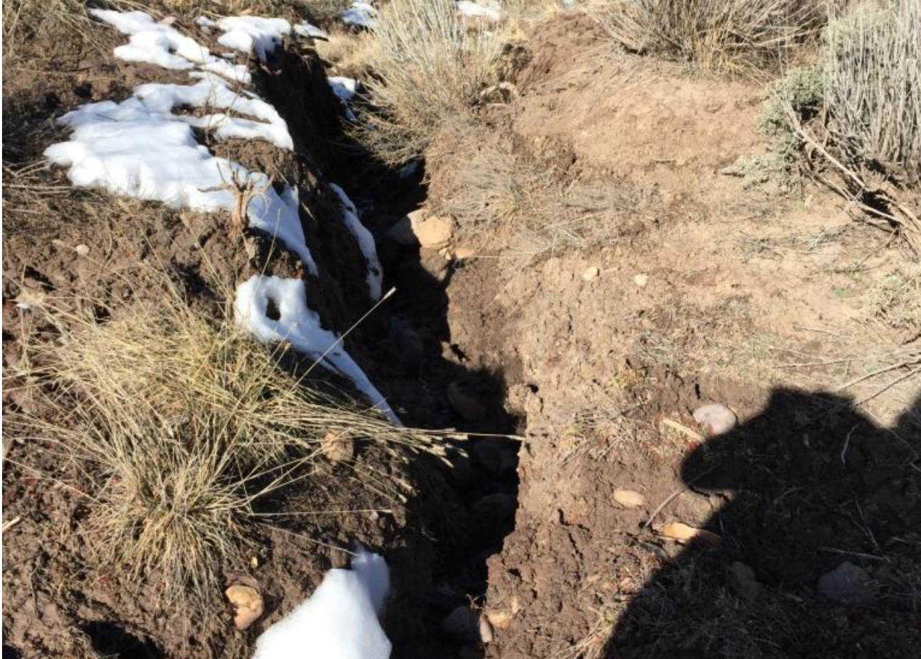
Photo 4. View of an erosional channel in northwestern corner of well pad that appears to be caused from stormwater overflow from silt trap in northern portion of project area (see Photo 5).
