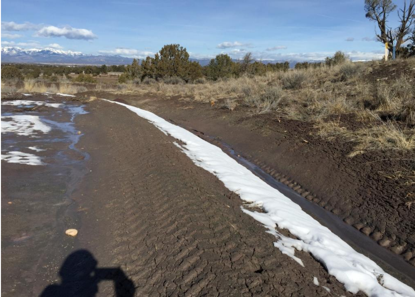
Photo 6. View of new berm and stormwater diversion along eastern edge of project area facing northward.
