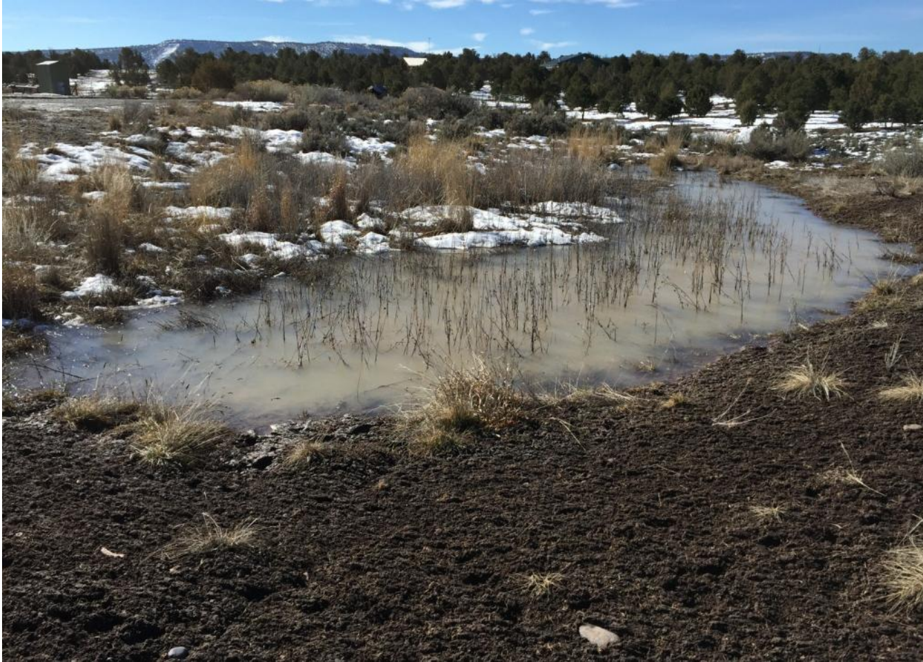
Photo 5. View of silt trap in northern portion of project area that appears to overflow and erode to the northwest (shown in background).
