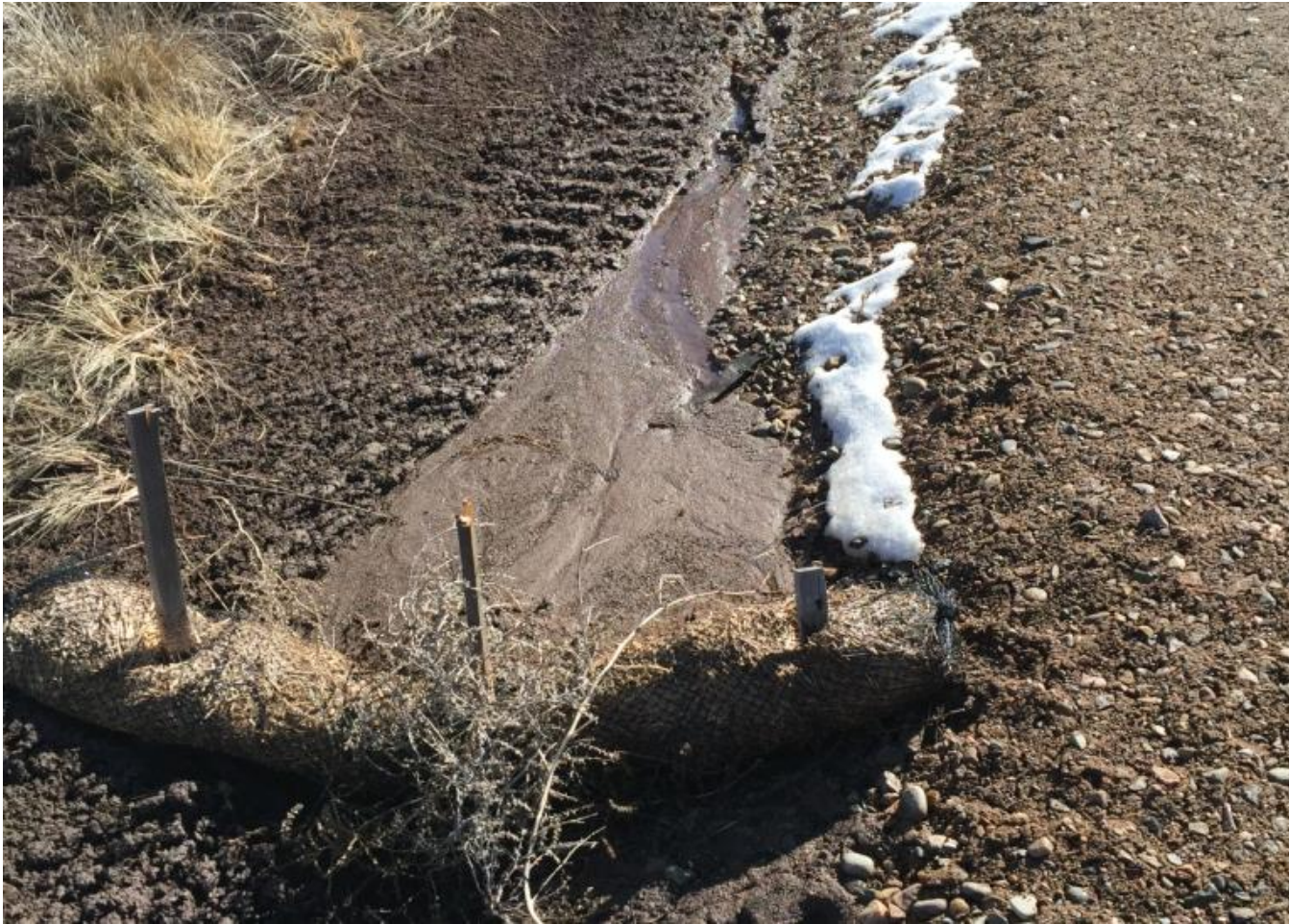
Photo 7. View of straw wattle along northern edge of access road that may not be sufficient to contain stormwater flows as it is almost full of sediment.
