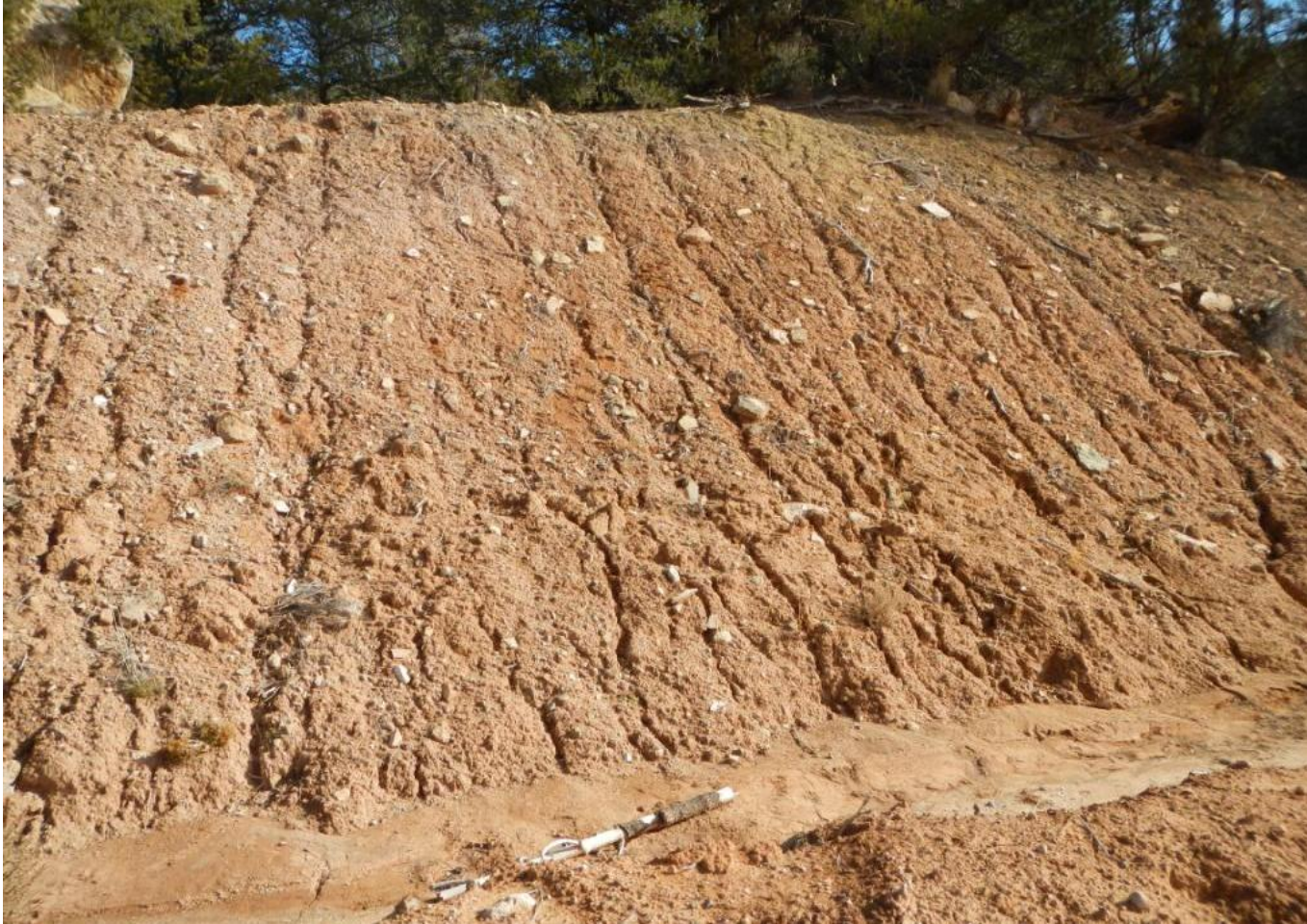
Photo 3. View of rill erosion and sediment deposition in and below a portion of the unprotected cut-slope in the eastern portion of the project area.
