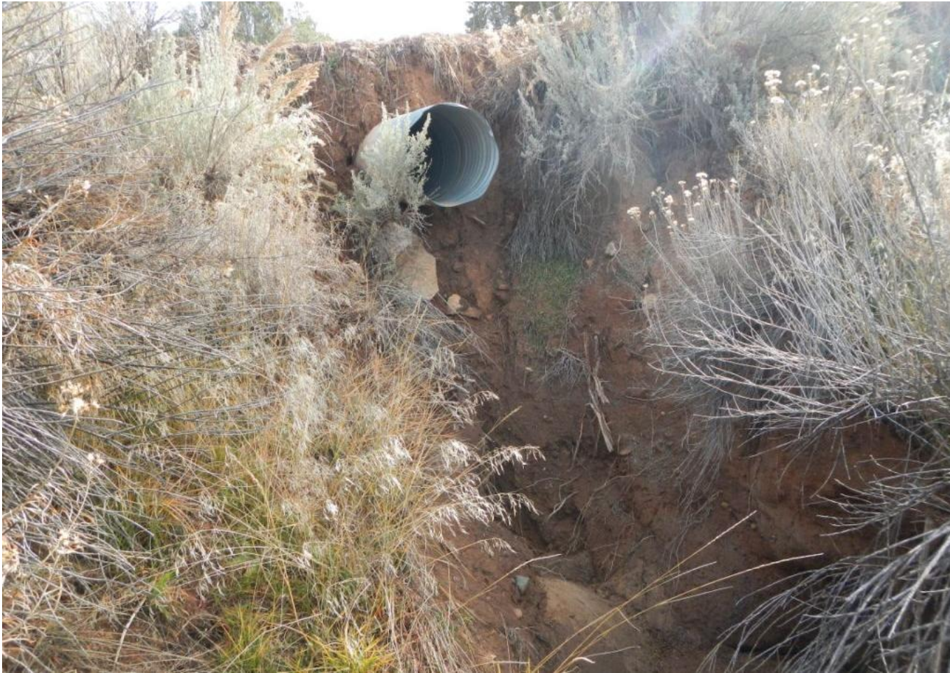
Photo 6. View of erosion at culvert outlet on the access road near the entrance to the well pad. Erosion from stormwater flows exiting the culvert appear to have eroded approximately 10 feet of soil.
