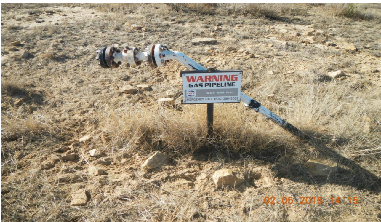
photo 2: Pipeline riser remains on the location. Lat/Long: 38.05236/-102.81947
