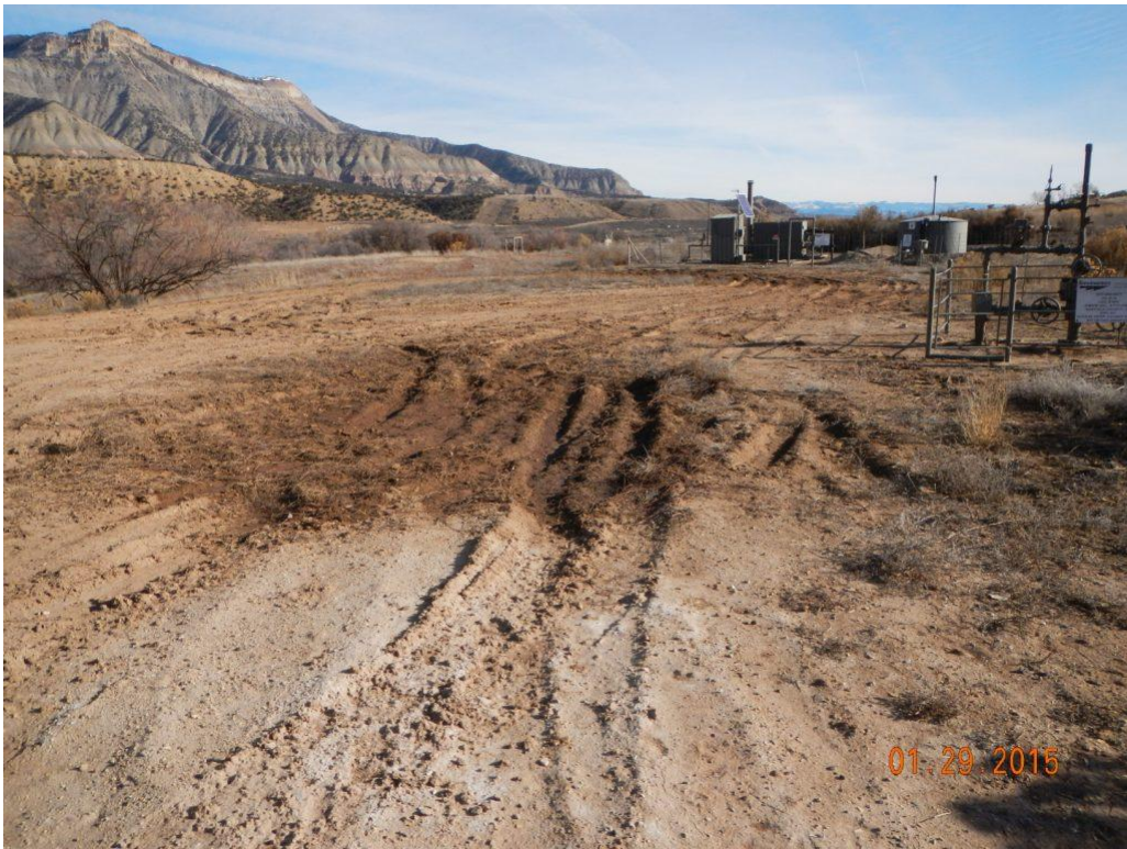
Subsidence on location.
