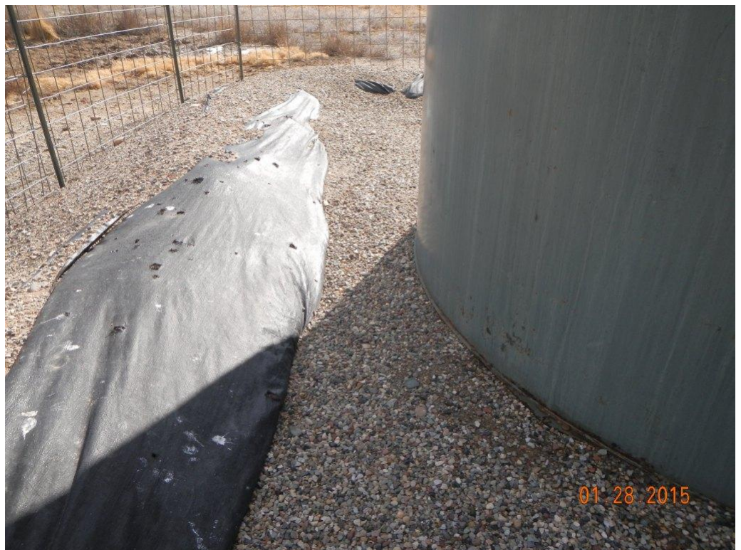
Liner in tank containment with holes.
