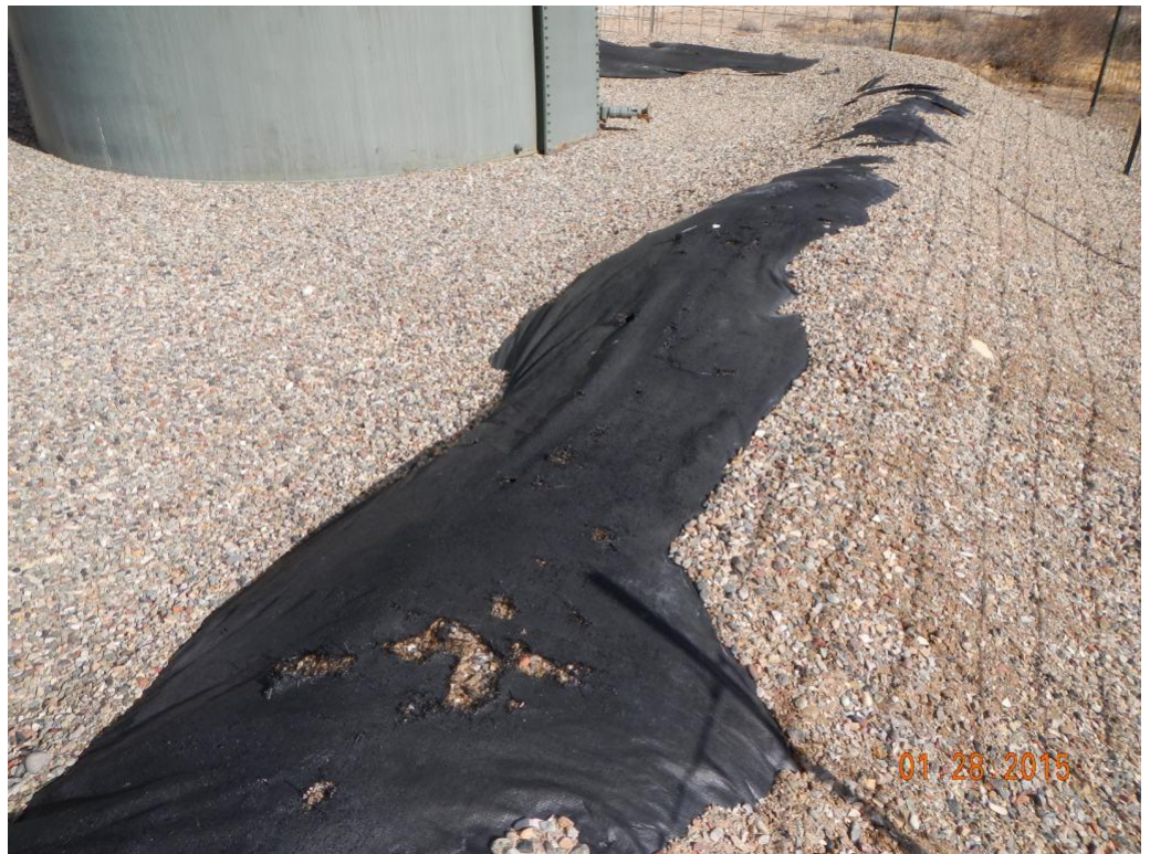
Liner in tank containment with holes.
