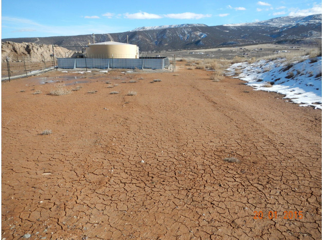
11. Approximately 40' x 70' on Southern side of separators area void of vegetation.
