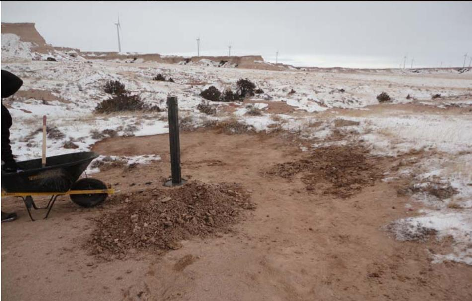
**Subject:** Photograph shows the steel riser completion for monitoring well, MW-2.
