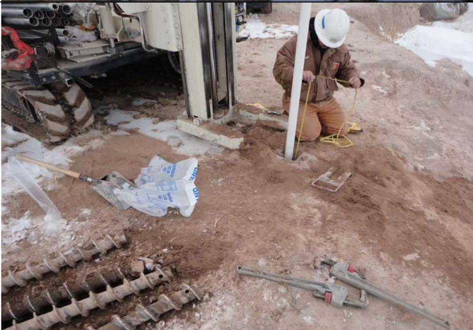
**Subject:** Site Services setting monitoring well MW-3 after augering down to 43 feet. The test hole collapsed back to 40 feet, which was where the well was set. A sand pack of 10-20 silica sand was placed around the screened interval in the well.
