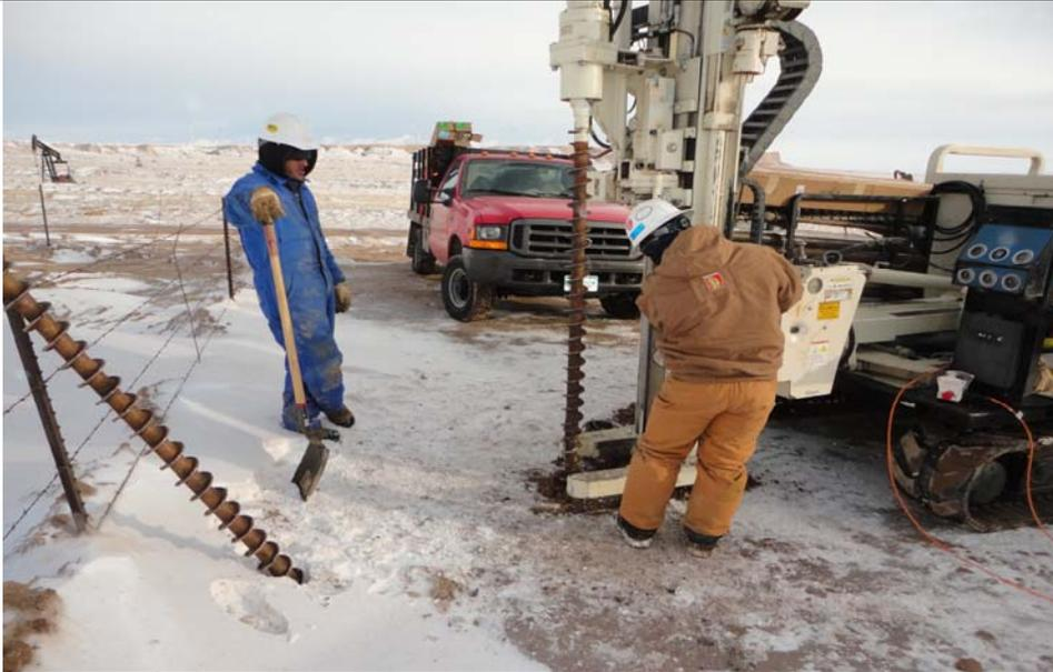
**Subject:** Site Services used 3-inch diameter solid stem augers to advance the test holes for the monitoring wells once probe refusal occurred. Photograph shows the test hole drilling for monitoring well MW-1 on the southeast side of the south produced water pit.
