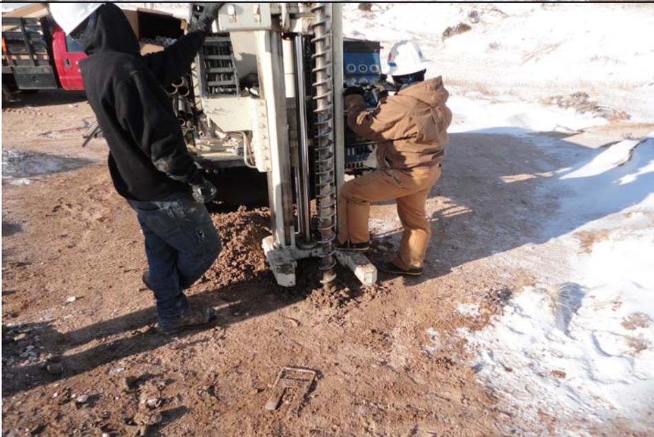
**Subject:** Site Services used 3-inch diameter augers to advance the test hole for MW-2 to 40 feet bsg.
