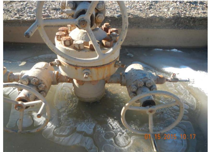
Three wall berm into cut wall allowing storm water and sediment into tank battery berm.
