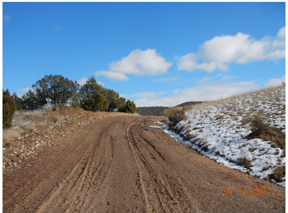
Rutting and erosion in roadway. Photo 2
