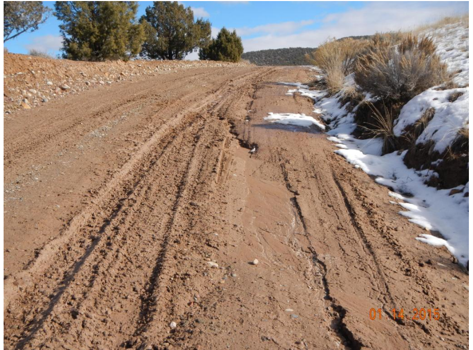
Rutting and erosion in roadway. Photo 1
