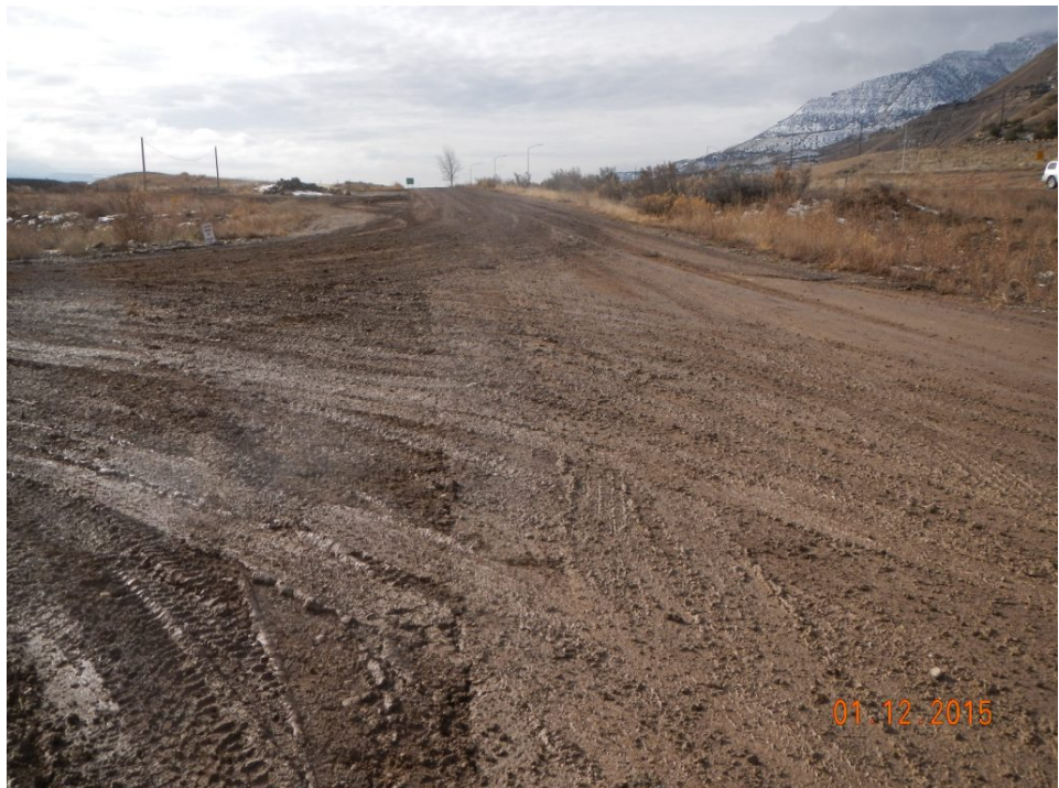
Vehicle tracking of mud onto pavement.
