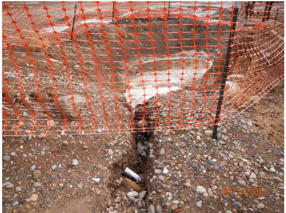
Erosion at retention pond at entrance. Trash in erosion rill.
