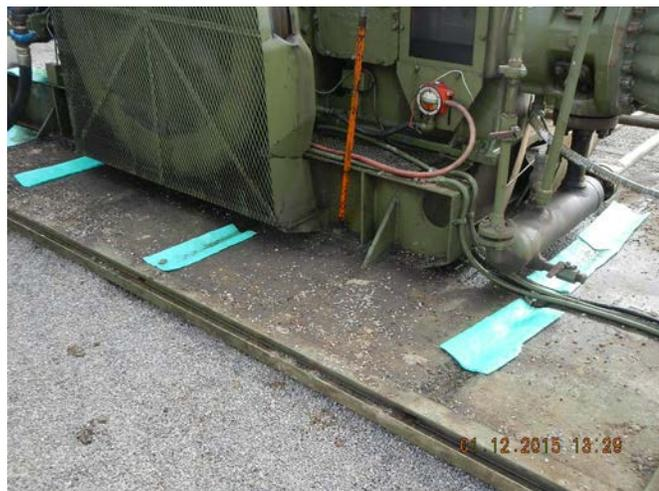
Horizontal heated separator drain plumbed to tank; Gravel added around equipment.
