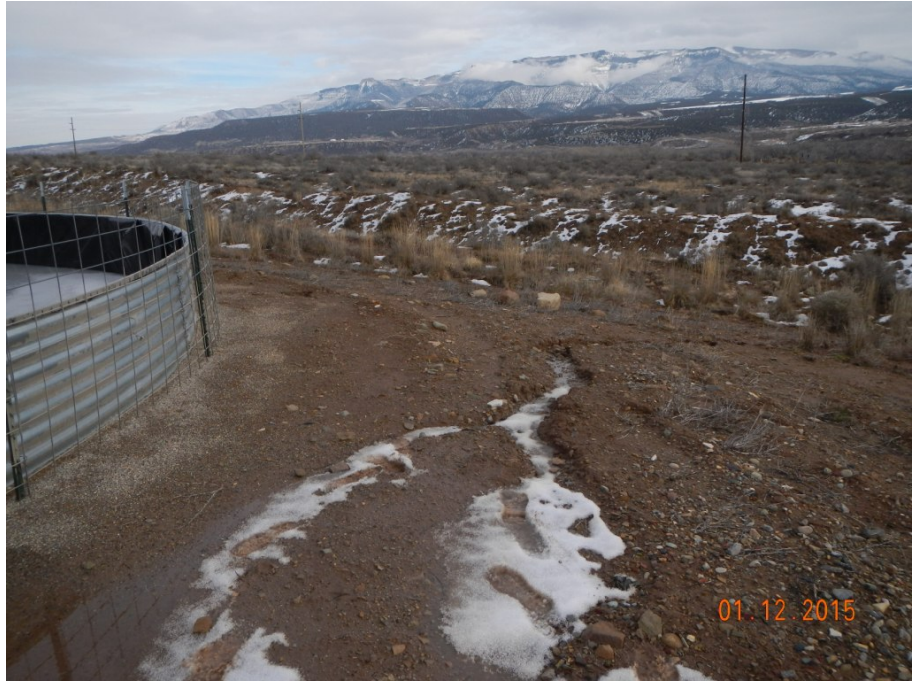
Erosion on SW side of location
